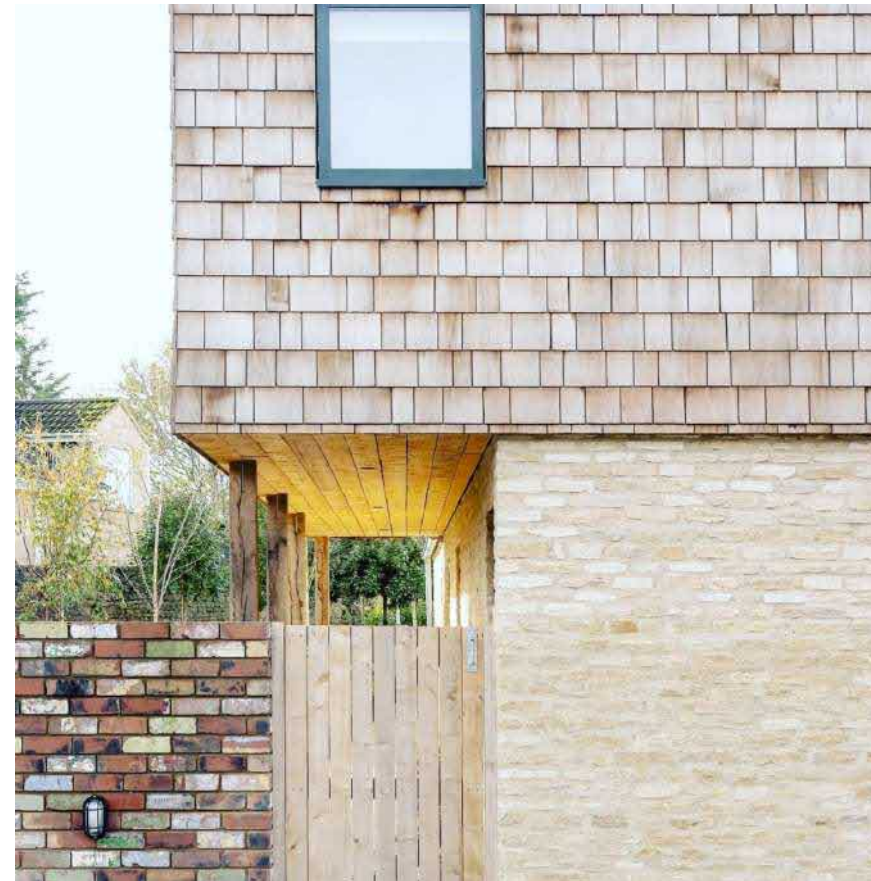
Light coloured brickwork with timber cladding at high level
