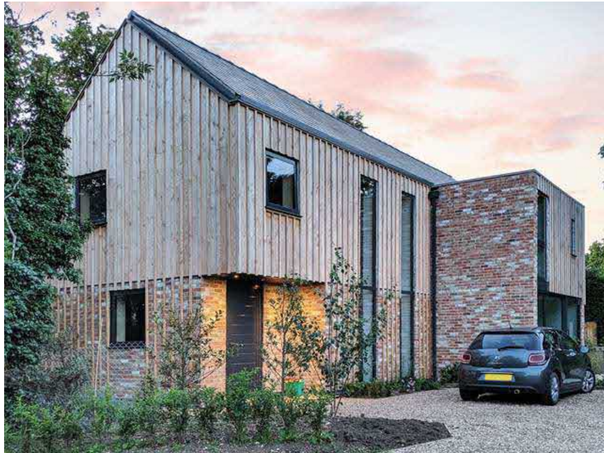
Brick base with timber cladding at high level, asymmetrical windows
