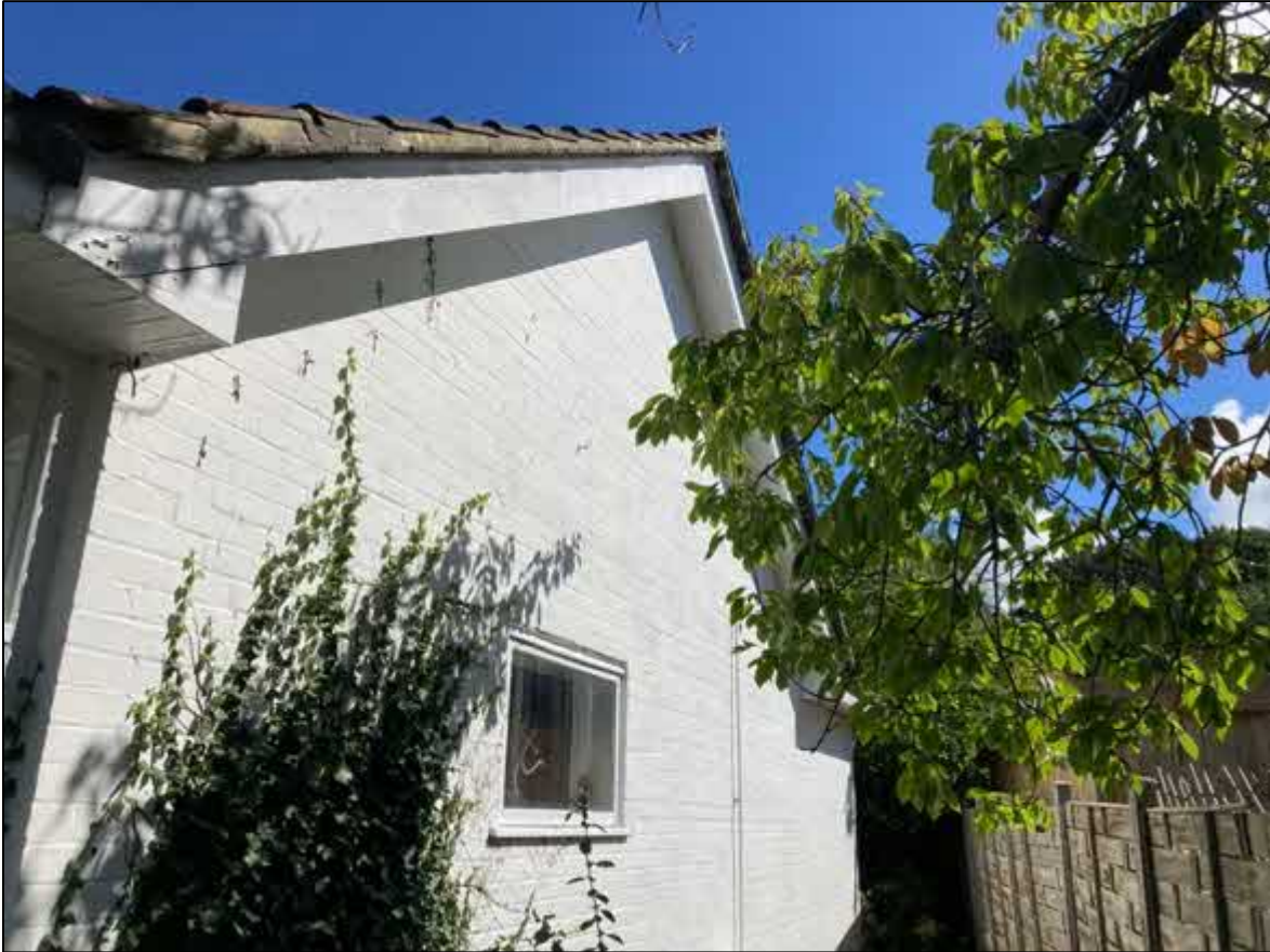
Photograph 3. Southern elevation of building.
