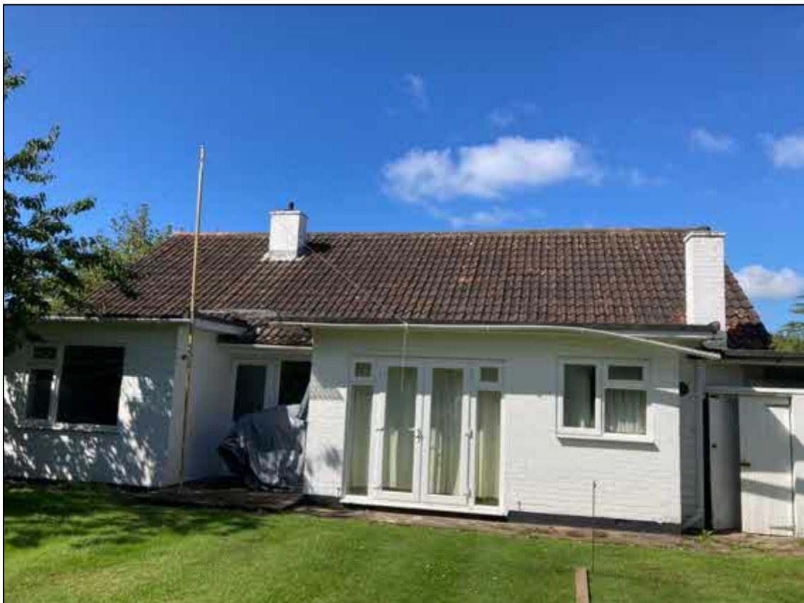
Photograph 2. Eastern elevation of building.
