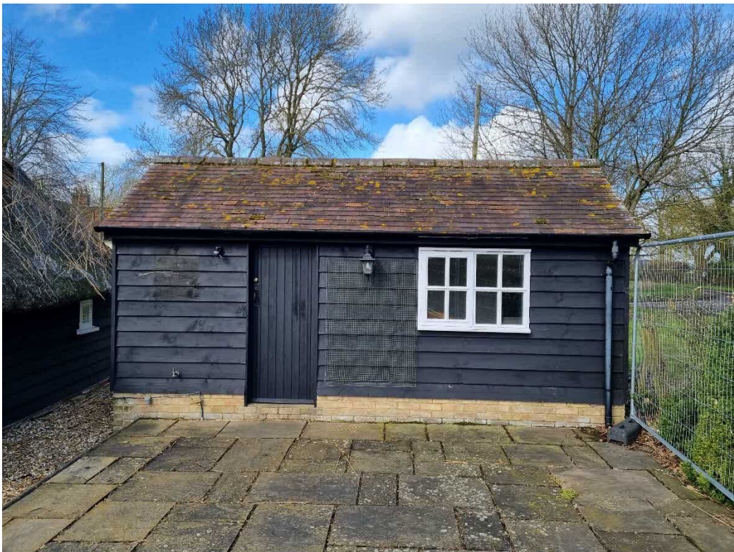
PHOTO 010 External view. Existing shed not affected by fire.
