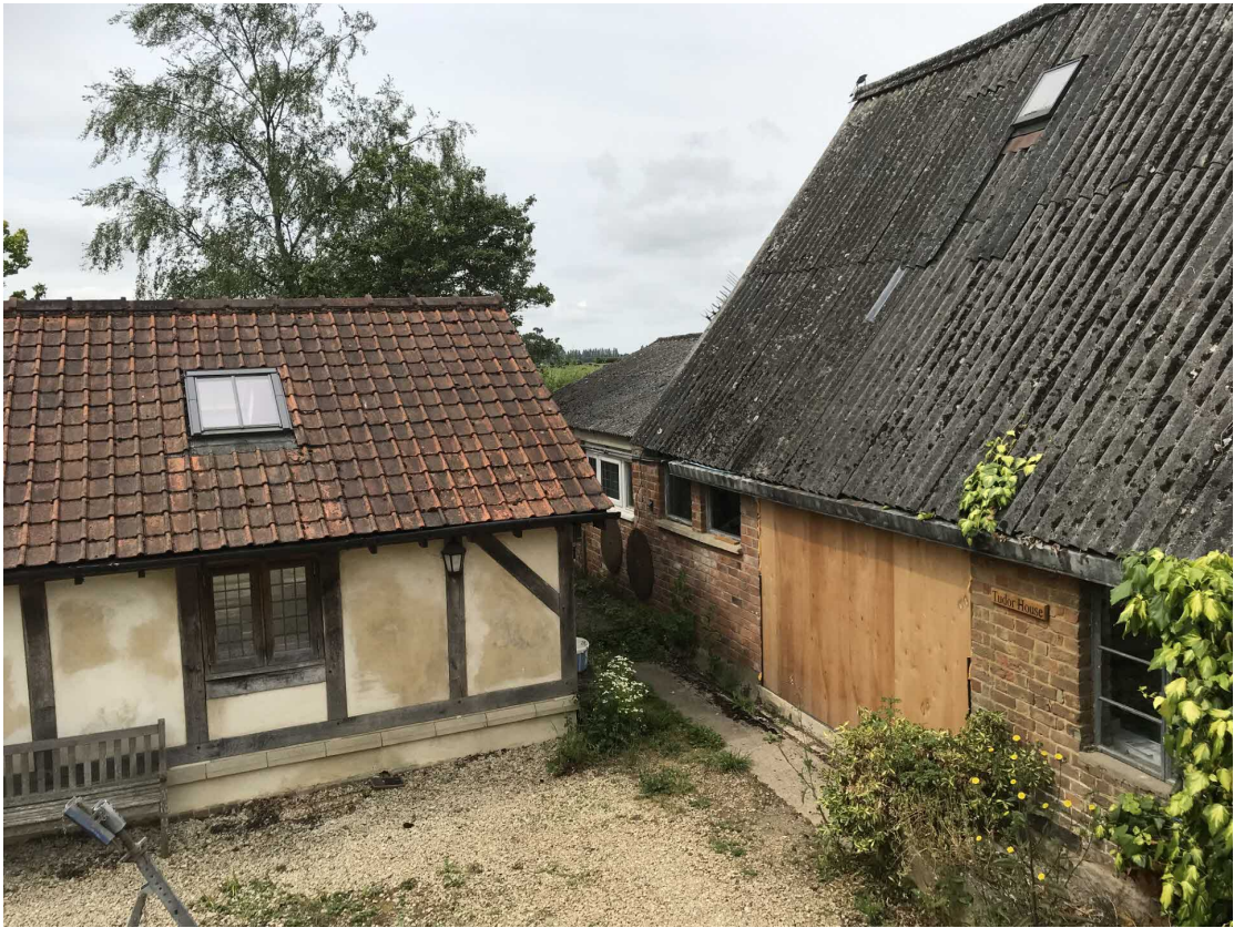
View from NE
