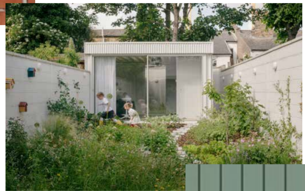
Green zinc cladding
