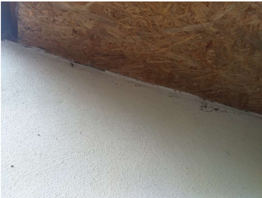
Tight seal between soffit and wall
