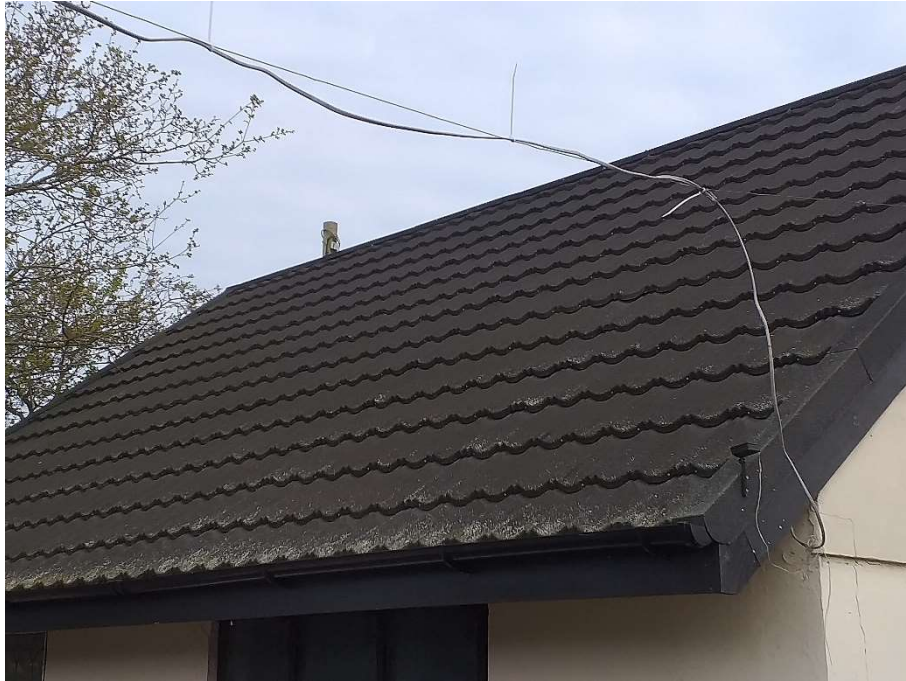
Tight seal on roof tiles
