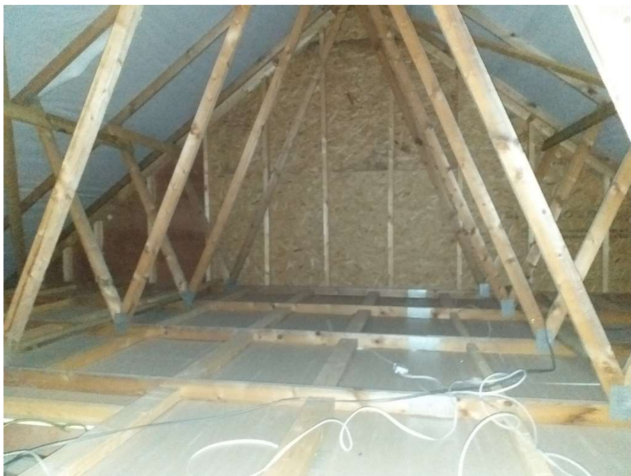
Roof void – no evidence of bats
