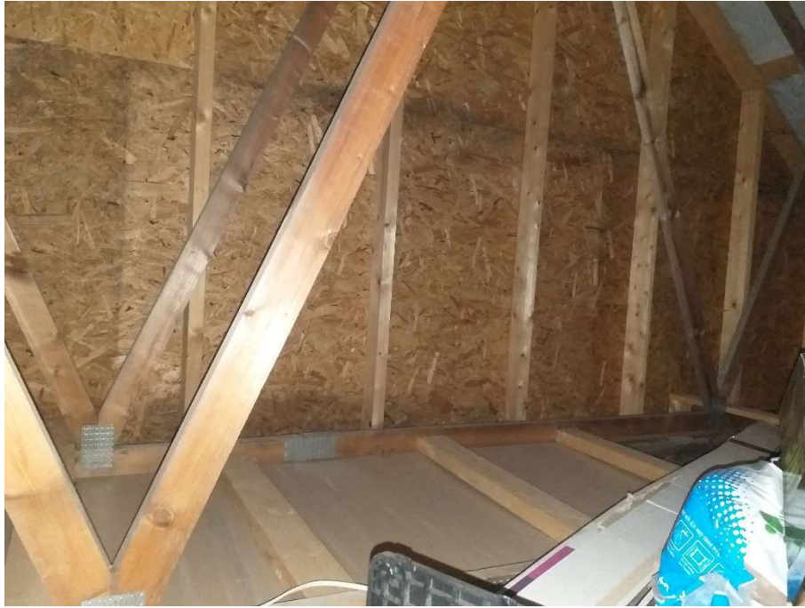
Roof void – no evidence of bats
