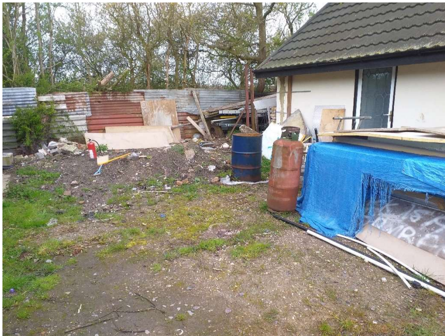
Yard located south of building
