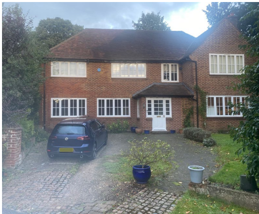
Fig 1. 7 The Grove front garden (West side)
