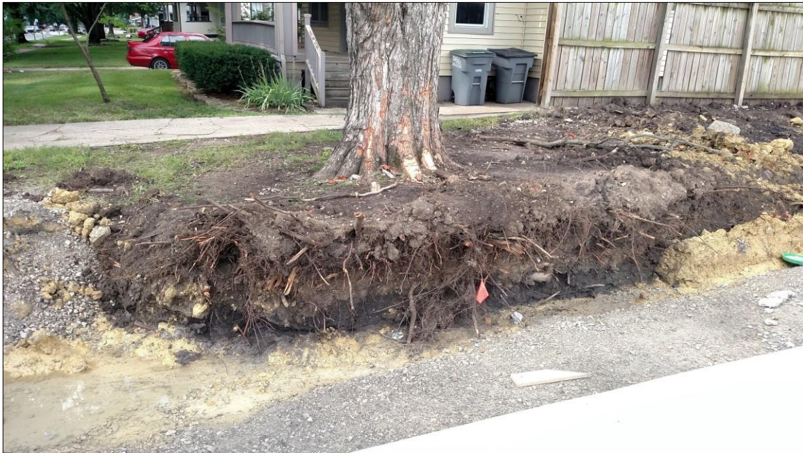
Fig. 1 Damage to roots can both kill and destabilise a tree. Planning work and care can avoid root damage
