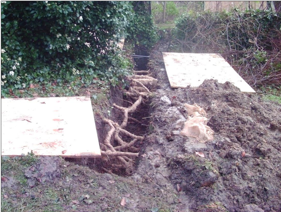
Fig. 2 Roots exposed, retained and protected during manual digging exercise
