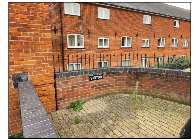
3. Existing Brick Wall with Iron Railings
