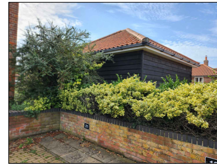
2. Existing Brick Retaining Wall
