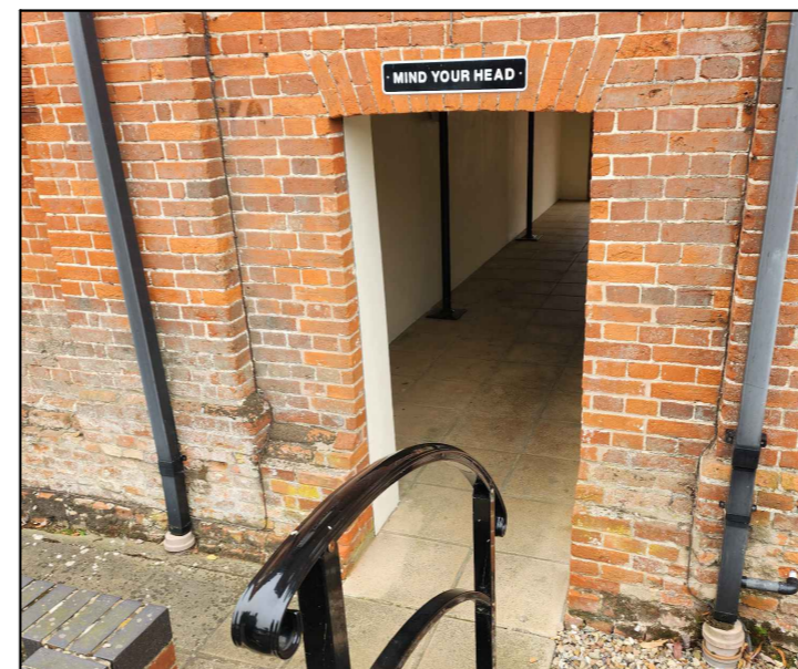
4. Existing Opening in Wall
