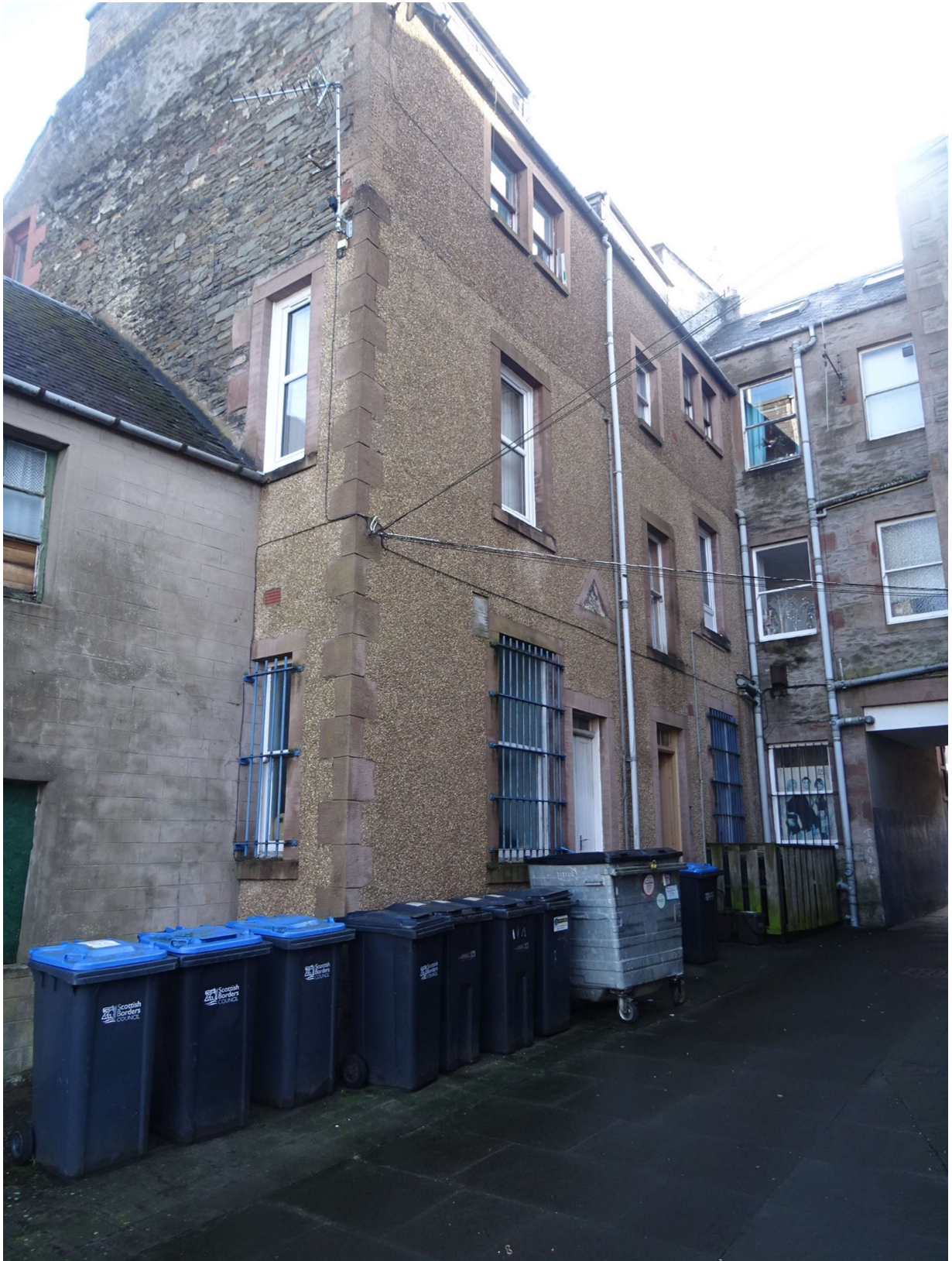
Rear Elevation to Close
