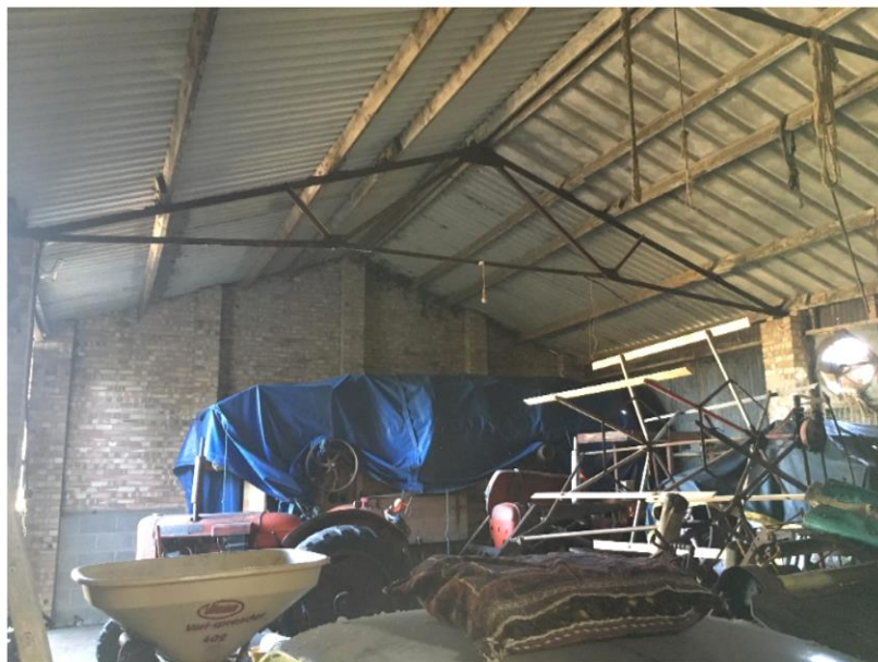
A1.2 Internal view showing roof and north gable
