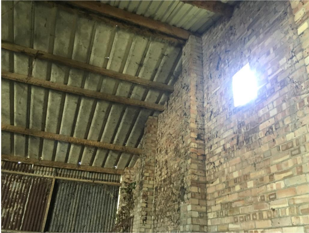
A1.3. Internal view of roof and South gable
