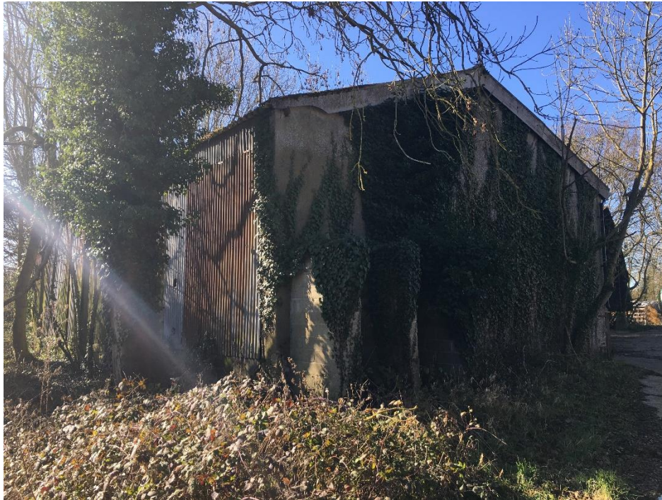
A1.1 North Gable with mature tree to East side
