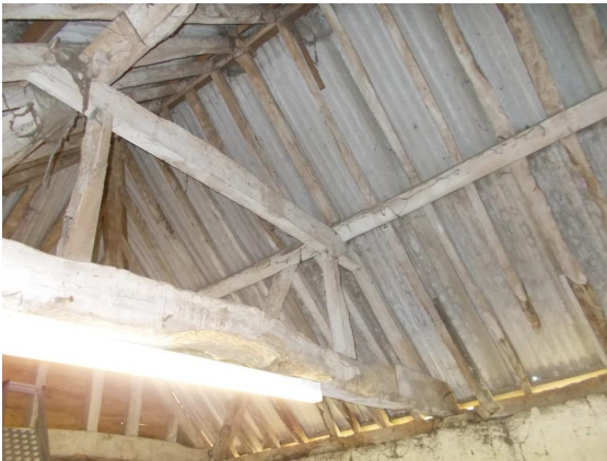
Photos show structural condition of internal trusses and rafters requiring extensive repair.
