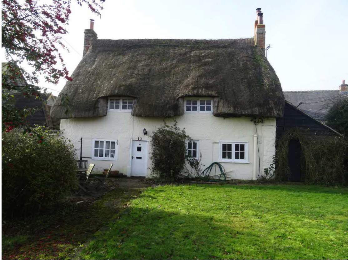
View of the Front Elevation
