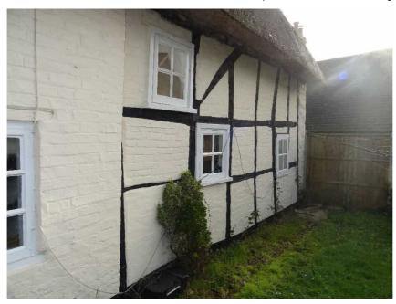
This is even more complicated where it appears that the gabled wall to the right hand side and small return to the rear is original and the brick section to the left of the rear return may have been rebuilt at some time and not tied to the stone so as the gabled wall sank the separation cracking has appeared.
