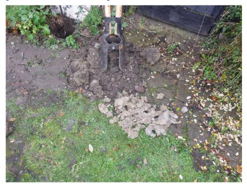
The trial hole was extended with a 50mm hand auger upto 2.3m below ground level with ground being a constant grey mottled clay.
