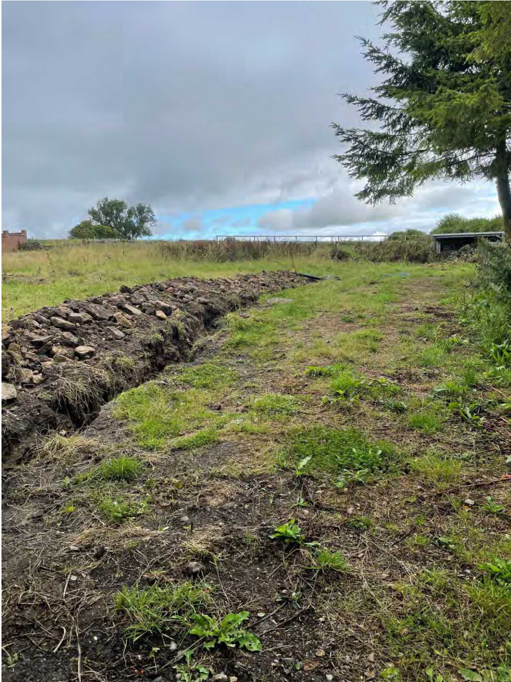
Photograph 1 – Drain system on the Southern border.
