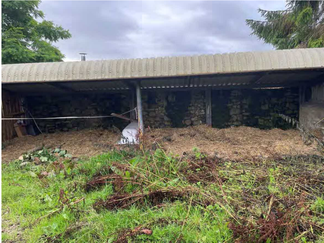
Photograph 2 – Stone, open fronted stables with metal roof on the Eastern boundary.
