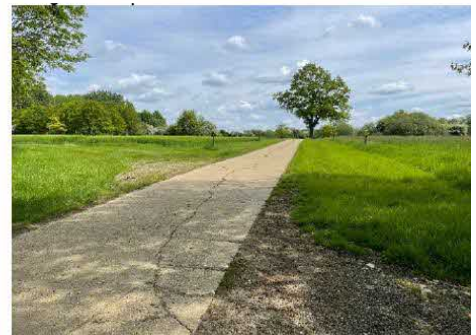
(iii) Concrete road
