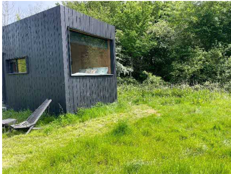
Example of already added cabin
