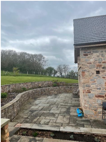
Picture: South view from east elevation
