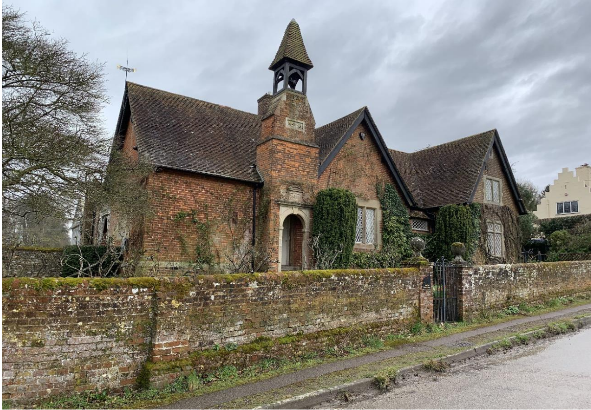
Fig. 1 – The Old School House; principal elevation facing Crows Camp Road.
