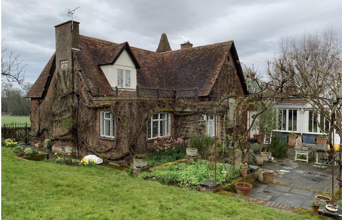
Fig. 3 – South-west facing elevation.
