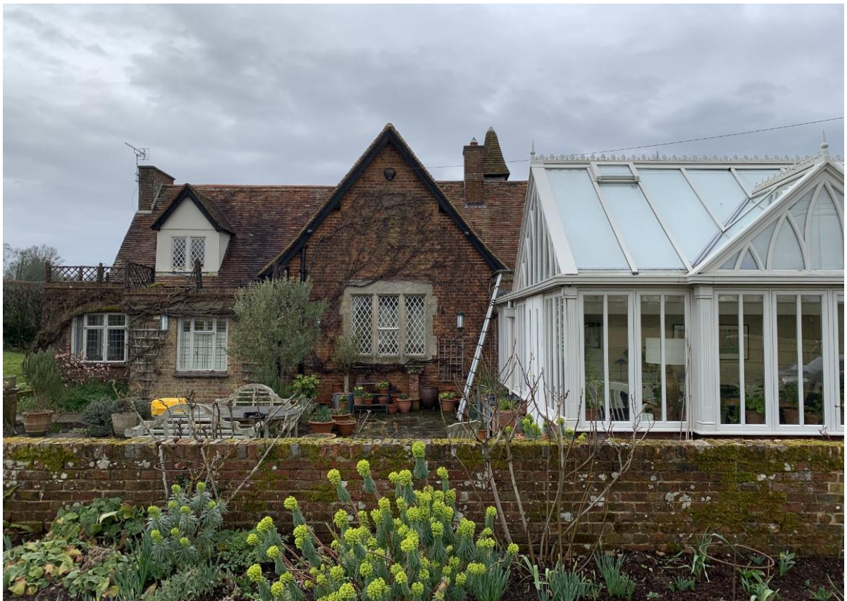
Fig. 2 – South facing rear elevation.
