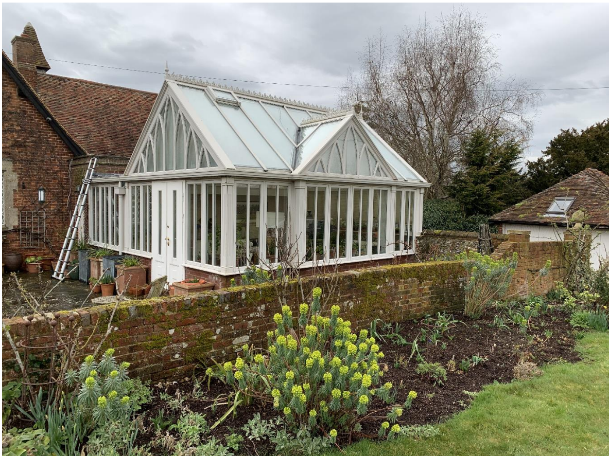
Fig. 11 – South-west facing elevation of existing conservatory to be replaced.
