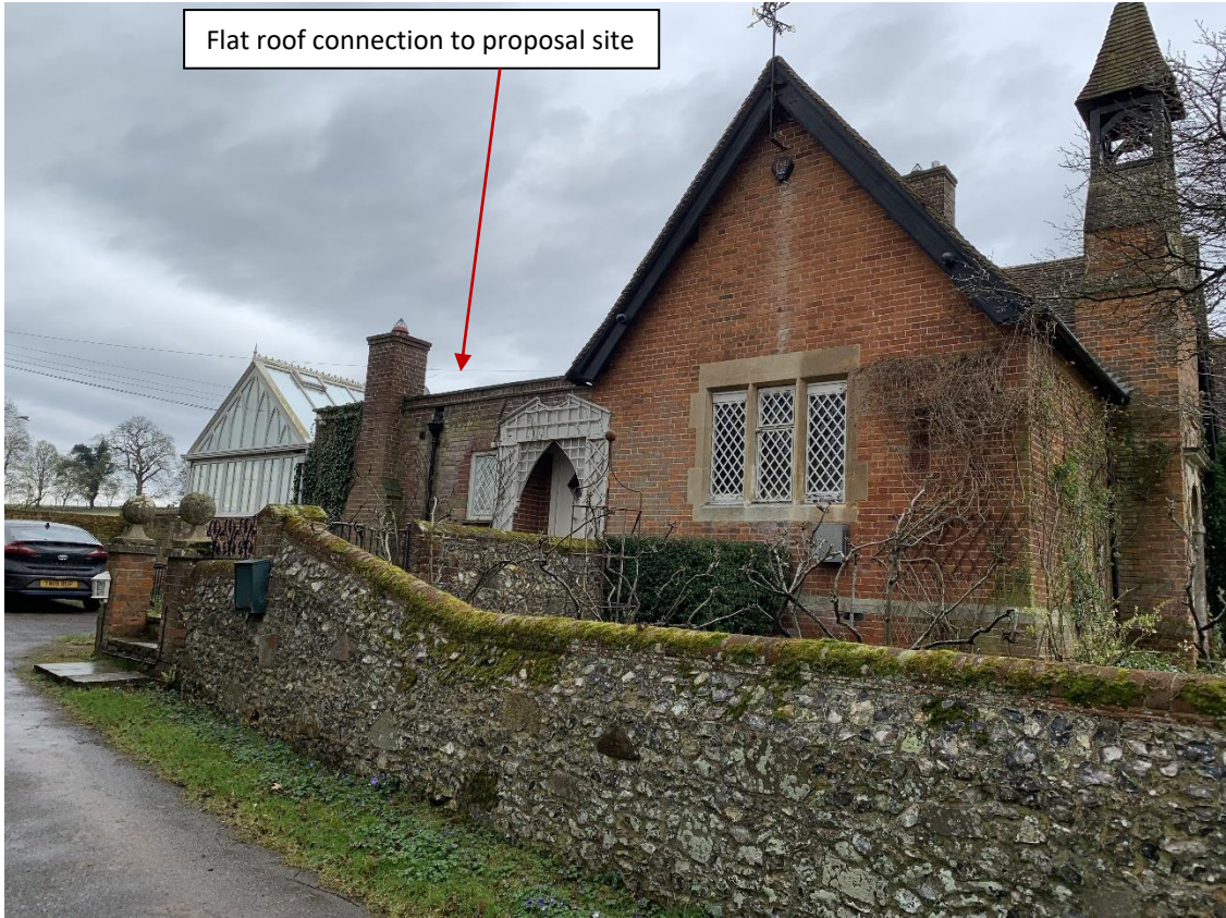
Fig. 12 – East facing / driveway elevation of existing conservatory to be replaced.
