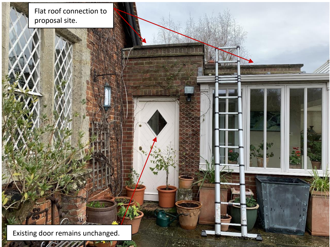
Fig. 13 – View of west elevation showing existing single door.
