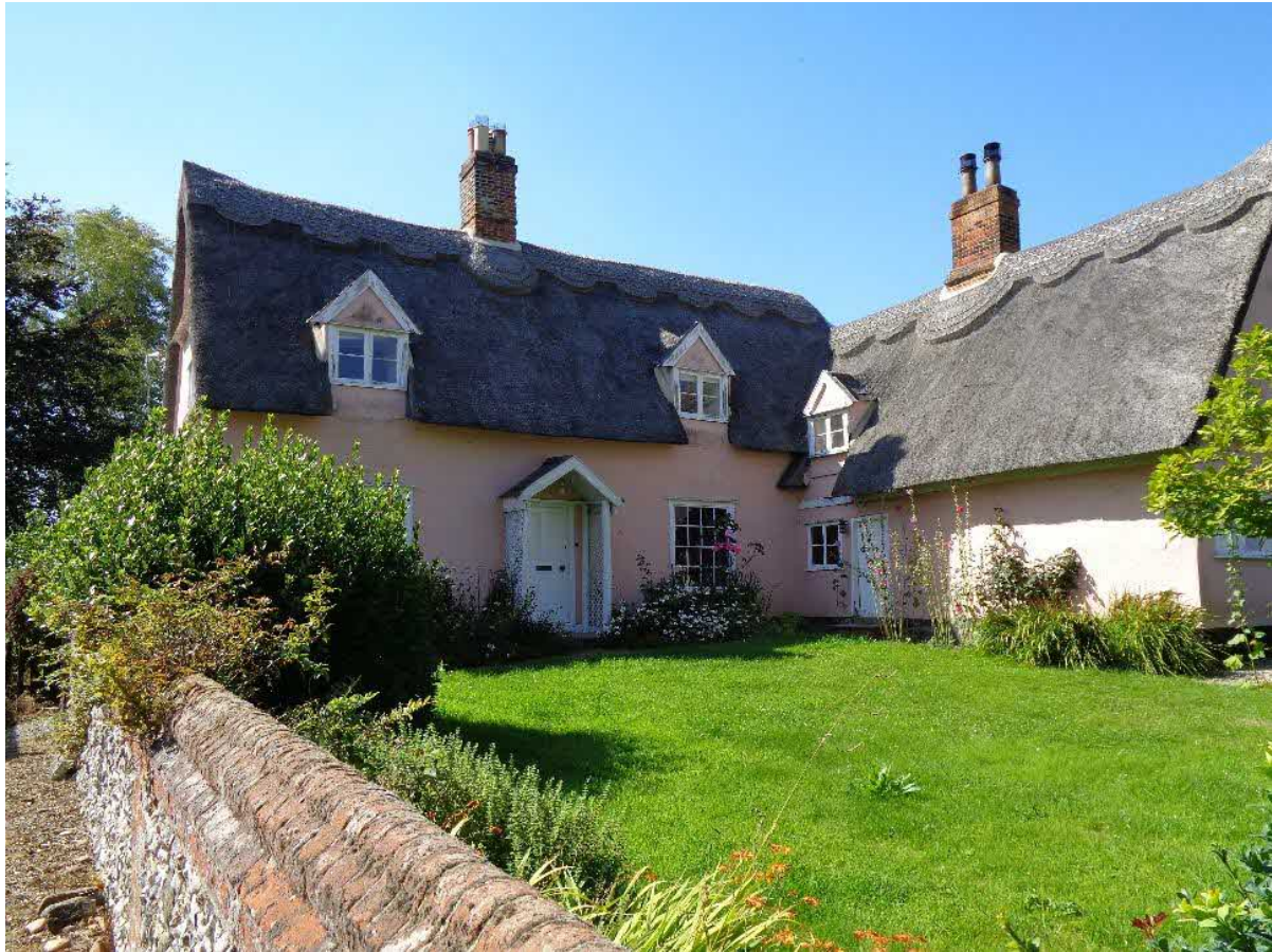
Principal elevation to the north
