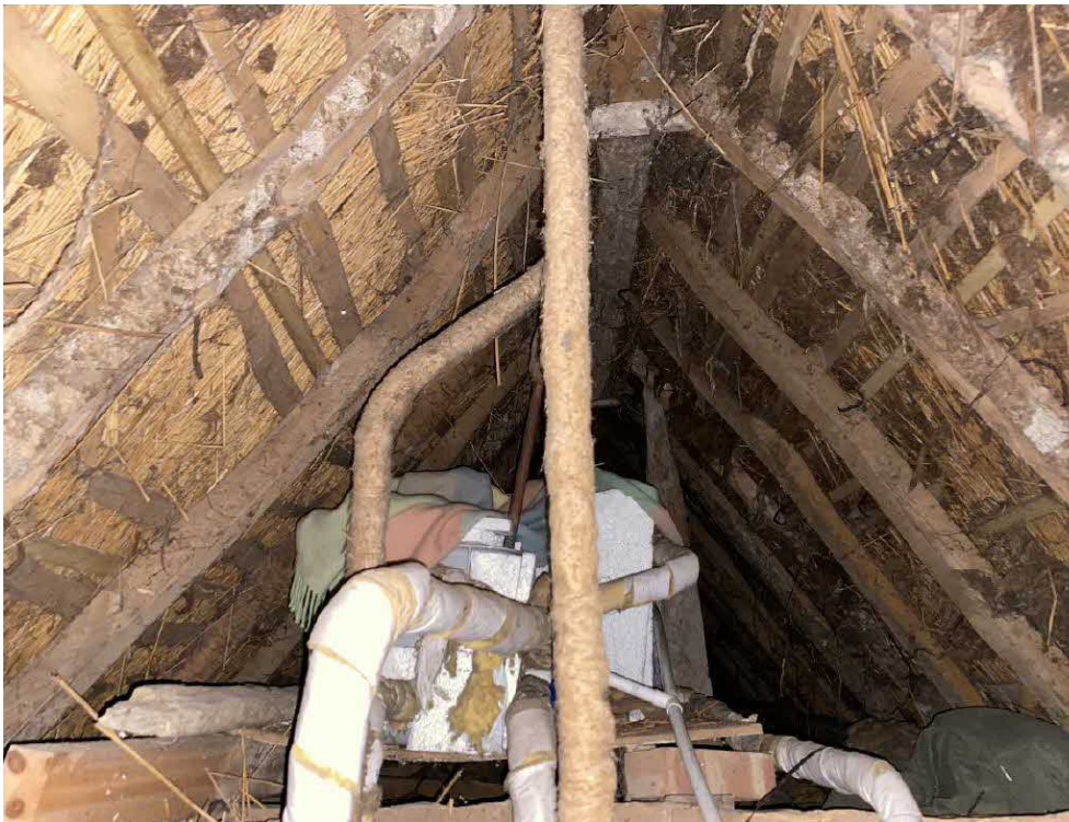
Photograph 79: Interior of attic of Building 1 (Andrew Firebrace Partnership, 2021)
