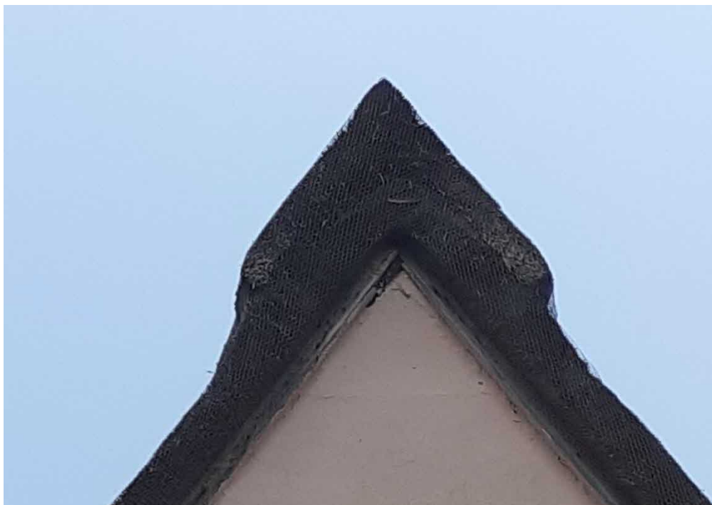
Photograph 23: Potential access point at the apex of the gabled roof, Building 1
