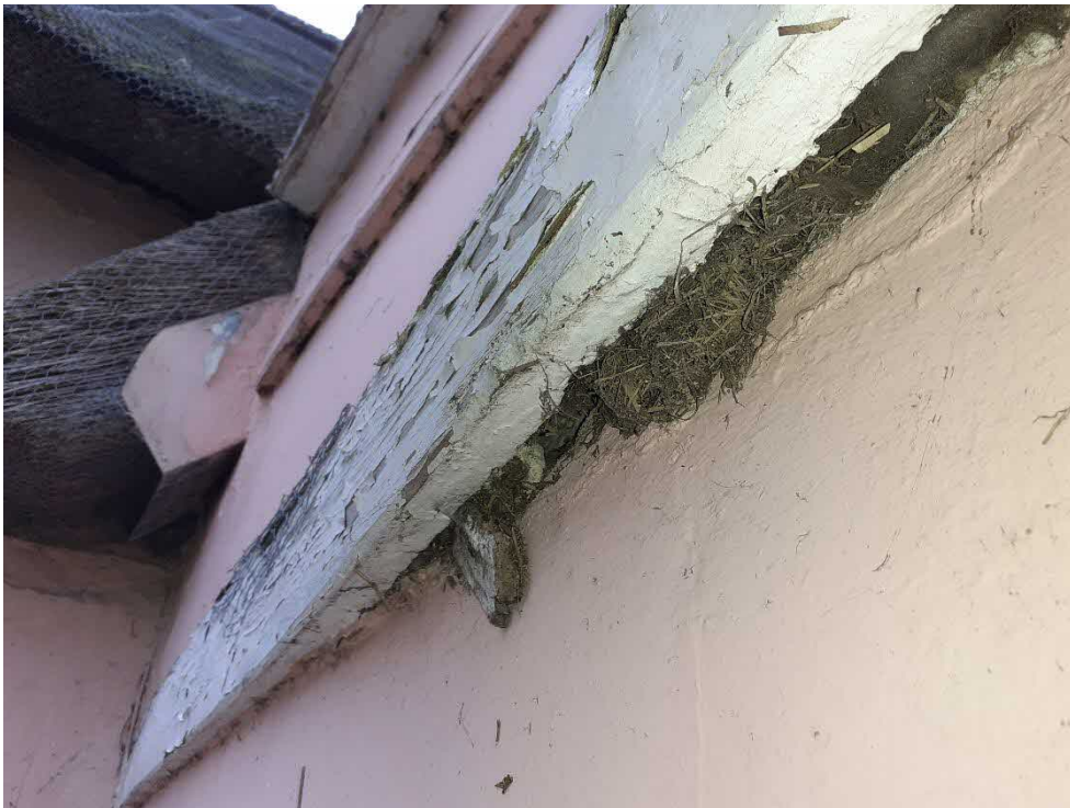
Photograph 65: Potential access point under the wooden beams of Building 1
