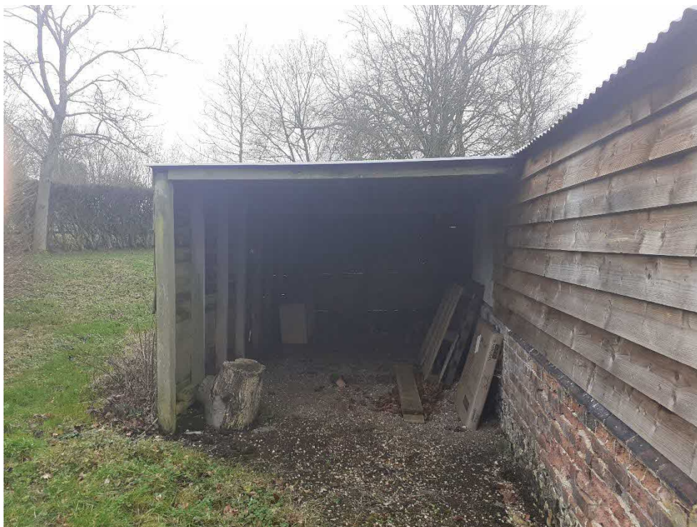
Photograph 31: Lean-to adjoining Building 2
