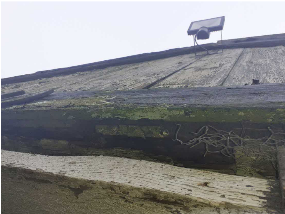
Photograph 34: Potential access points under the wooden panels of Building 2
