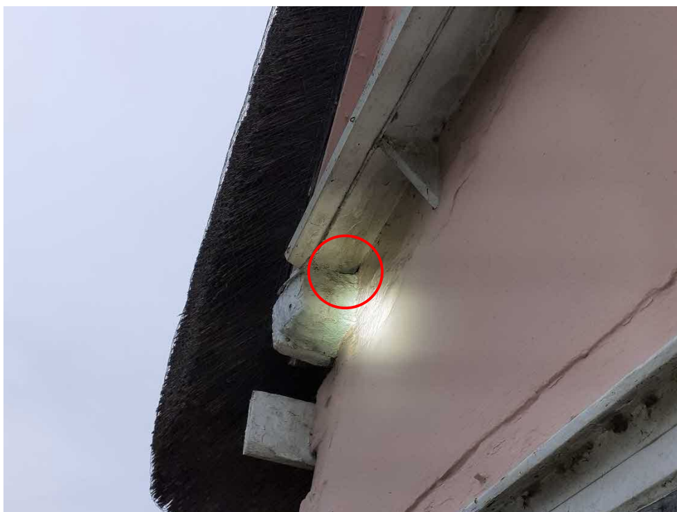
Photograph 24: Potential access point between the wooden beams of Building 1
