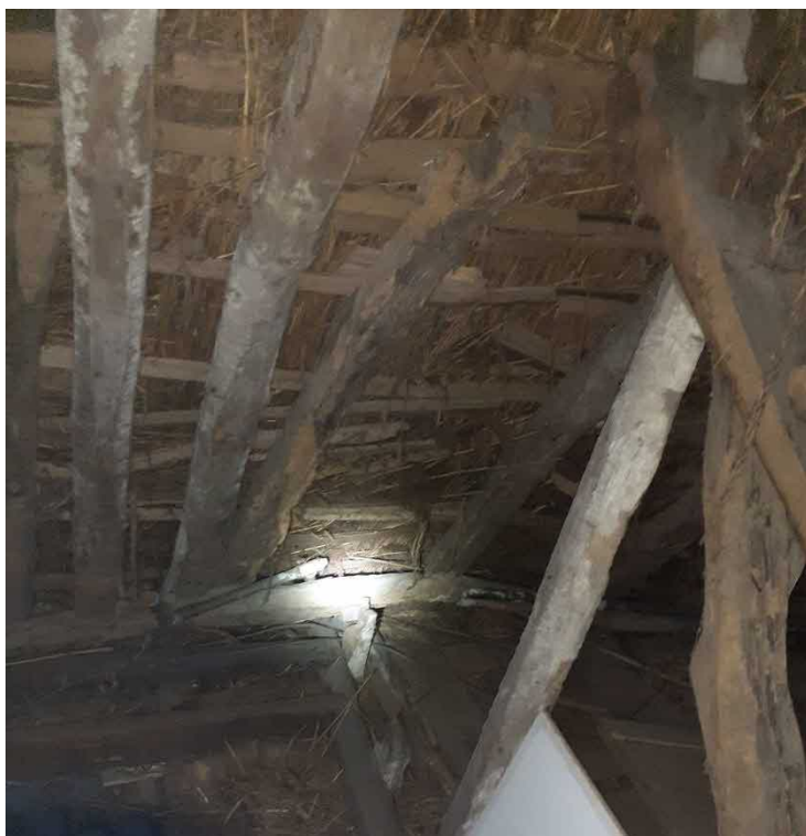
Photograph 28: Interior of attic of Building 1
