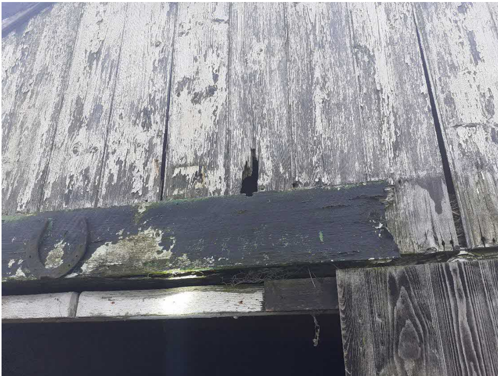
Photograph 33: Potential access points between the wooden panels of Building 2
