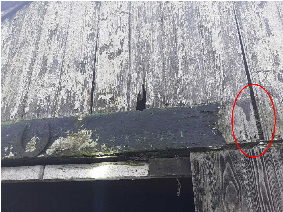
Photograph 40: Bird nest found in the wall cavity of Building 2
