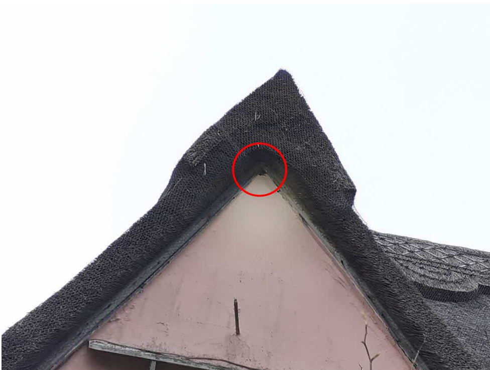
Photograph 22: Potential access point at the apex of the gabled roof, Building 1
