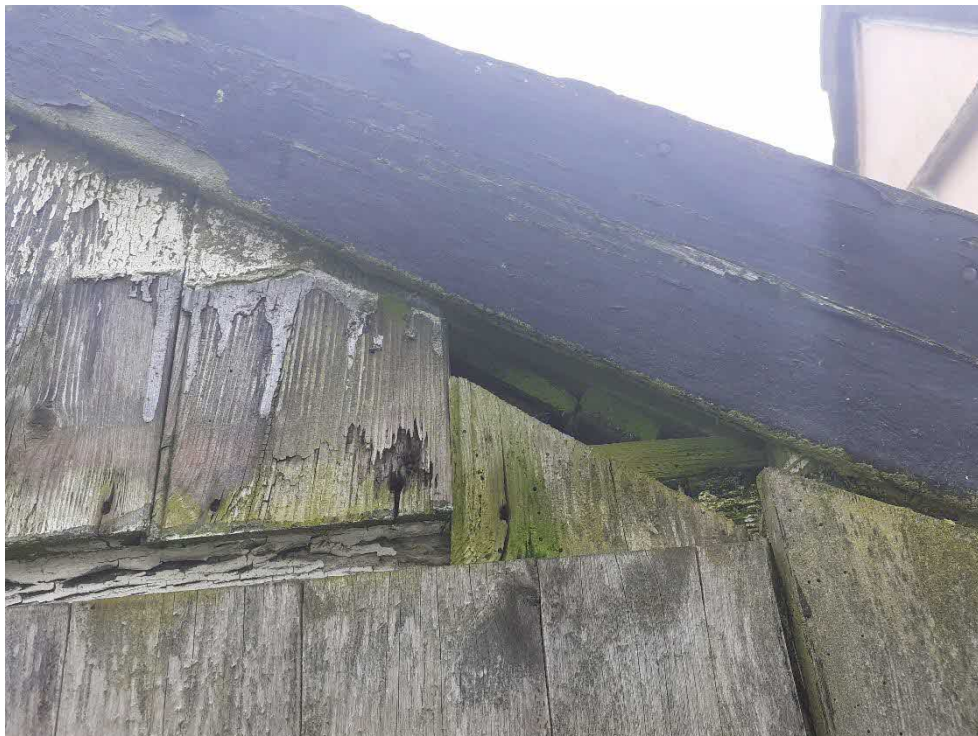
Photograph 32: Potential access points between the wooden panels of Building 2
