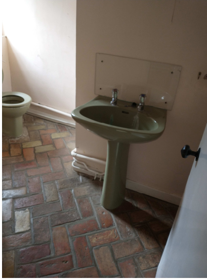
Figures 4.1 – herringbone bricks with cement mortar to be removed
