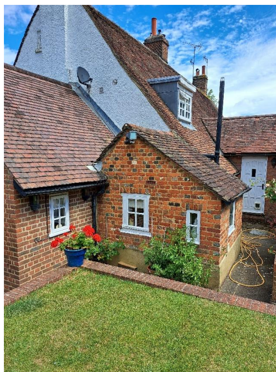
Rear Ground Floor Window (RW1)
