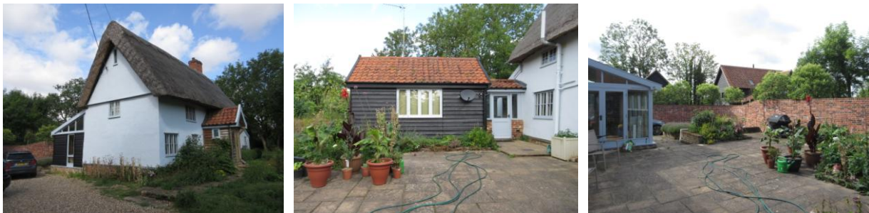
Left: looking W showing SE elevation of cottage and lean to garden room; Centre: looking NW from paved courtyard to rear of cottage showing study and link; Right: looking SE from outside study showing courtyard, brick boundary wall and Hart Barn beyond
