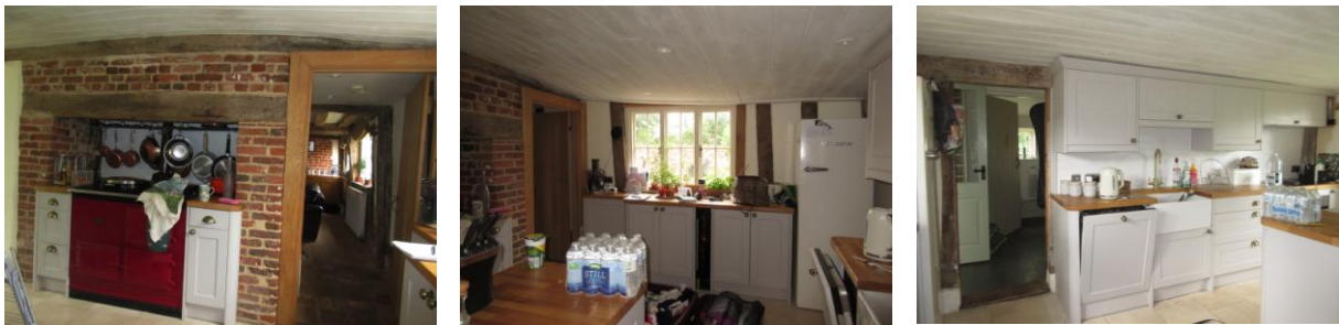
Left: fireplace in SE wall and door to living room; Centre: looking SW showing boarded ceiling and 20th century casement inserted into SW wall; Right: looking NW showing door to utility room (in lean to extension) with exposed section of wall plate above
