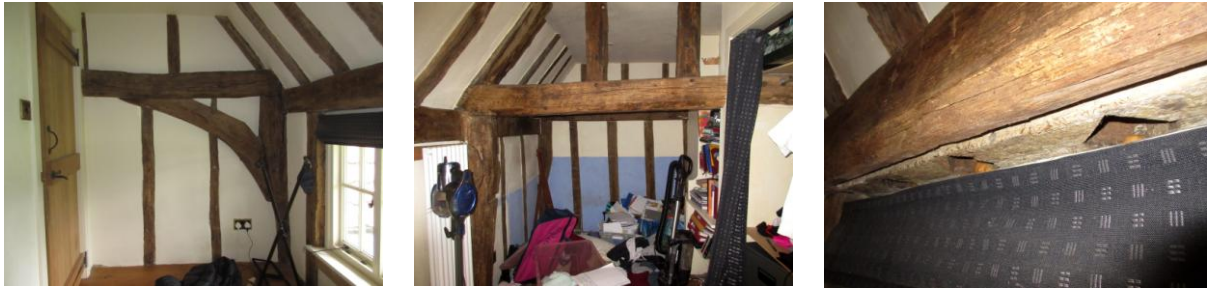
Bedroom 4: cranked arch brace at NE end of tie beam looking NW; Centre: looking SE showing open studs above tie beam with jowelled main post; Right: diamond mullion mortices above NE window
