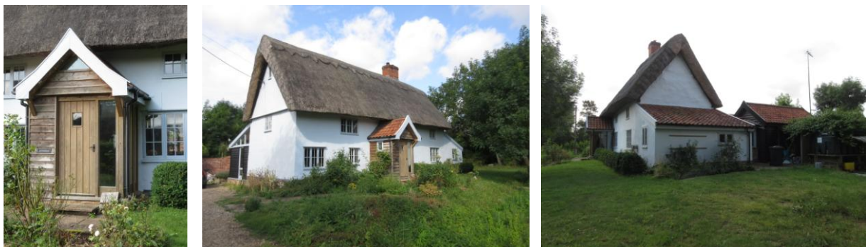
Left: detail of porch looking SW; Centre: looking NW; Right: NW elevation showing lean to extension and linked 21st century single storey study/bedroom (right) with pantile roof
