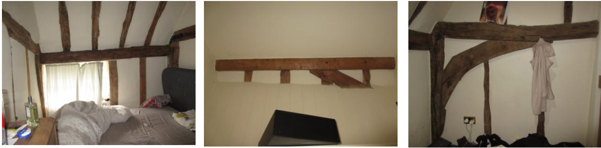
Left: Bedroom 2 looking SW; Centre: Bedroom 2 looking NE showing purlin and top of cranked wind brace above partition wall; Right: Bedroom 3 looking NW showing cranked arch brace beneath tie beam
