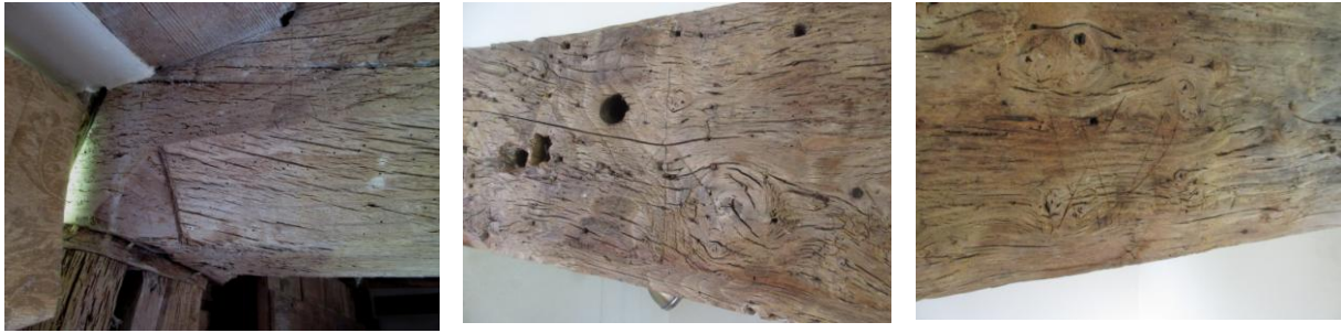
Left: stepped stop at end of broad chamfer on cross axial beam; Centre & Right: supersticious apotropaic or witch marks on bressumer face
