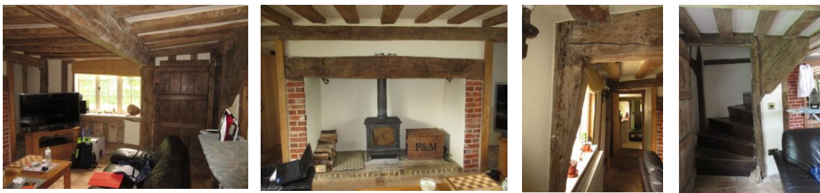
Left to Right: looking NE showing plank and batten front door; fireplace looking NW; jowelled main post in SW wall; looking SE showing staircase in SE corner of living room
