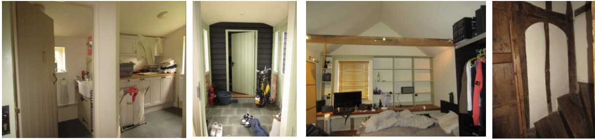
Left to Right: utility room looking NW; glazed link looking SW; interior of study bedroom looking SW; 3-centred arch of former cross passage in NE wall at foot of inserted staircase
