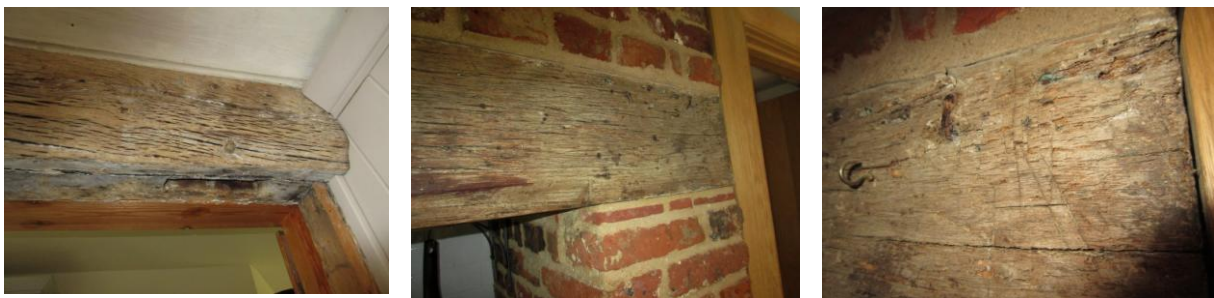
Left: empty mortice in underside of NW wall plate, removed to form doorway in former external wall; Centre: detail of bressumer showing chamfer with flat stop; Right: apotropaic marks incised on face of bressumer
