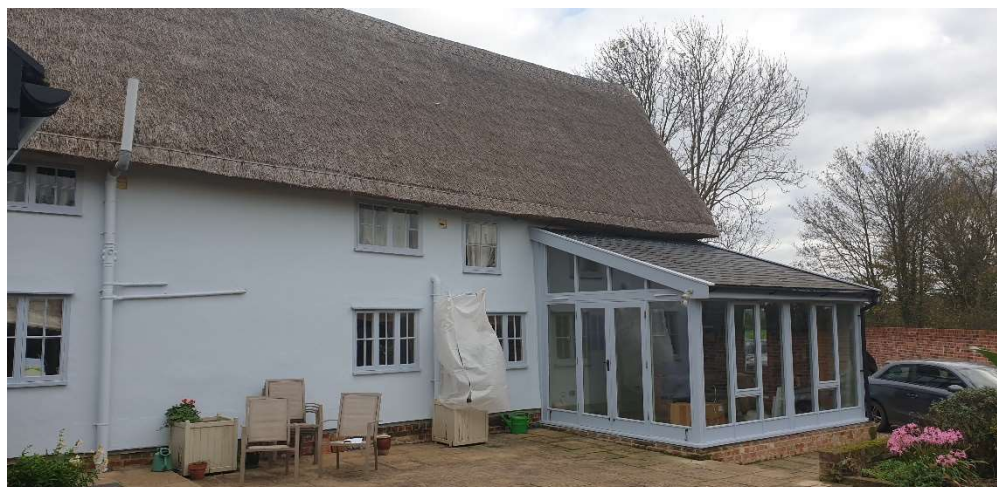
View of the rear from the west
