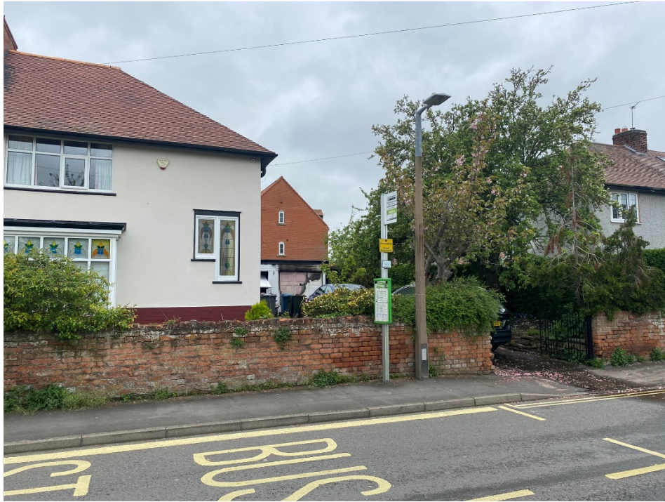
Existing front view of No 6 Cherry Street
