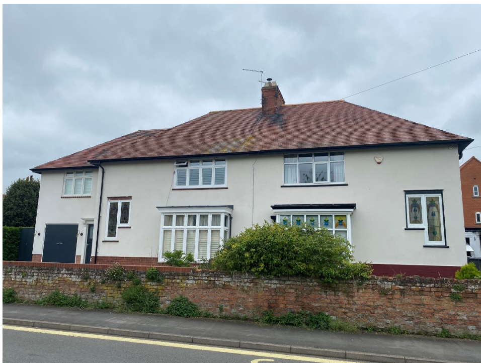
Existing front view of No 6 Cherry Street
