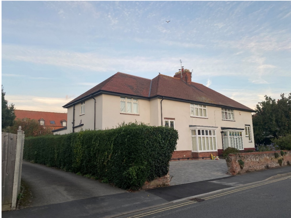
Existing front view of No 8 Cherry Street approved widened wall and dropped kerb.
