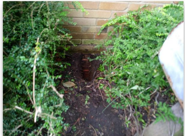
Fig 1.2: Trial Hole 1 Location
