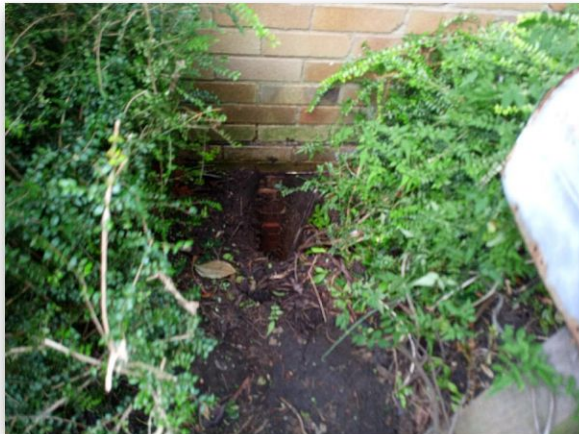
Fig 1.3: Trial Hole 1 Footing
