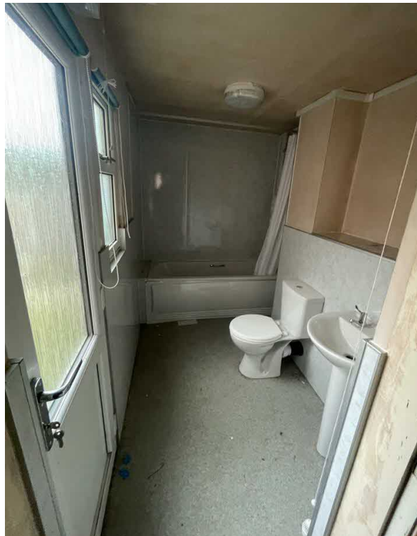
Photograph 4. Ground Floor Bathroom
