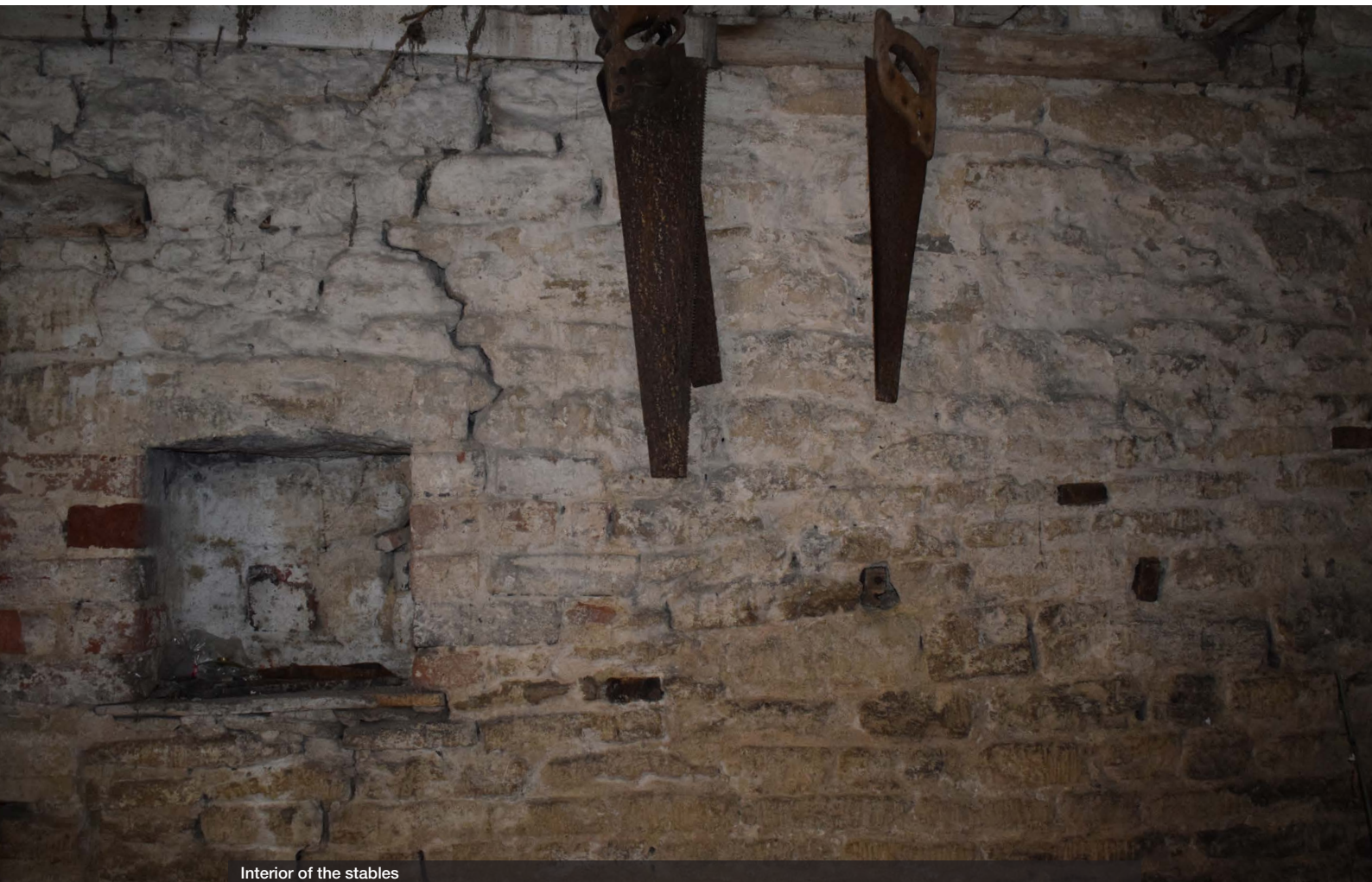
Interior of the stables
