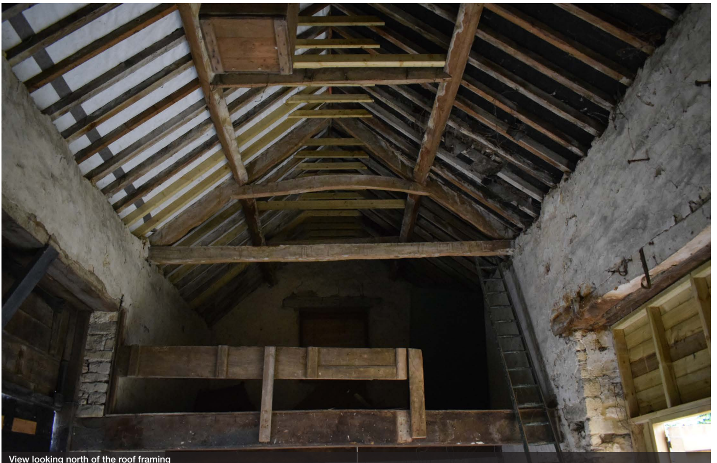
View looking north of the roof framing
