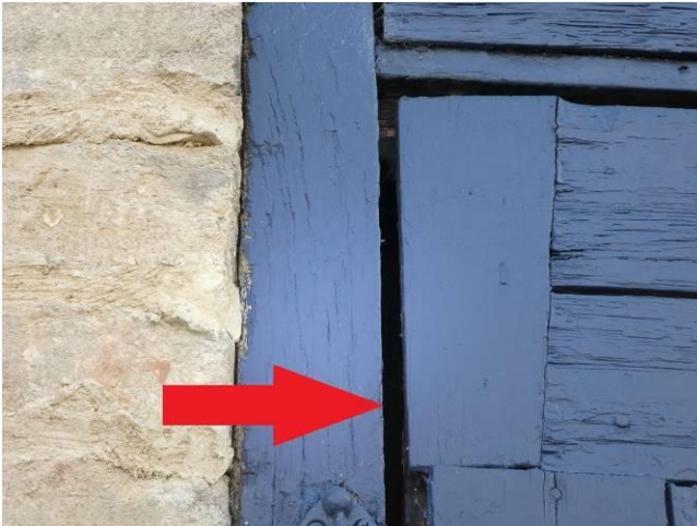
Photo 5 – Gaps at the side of the front elevation barn door, and, Photo 6 – Inside Lords Farm Barn
