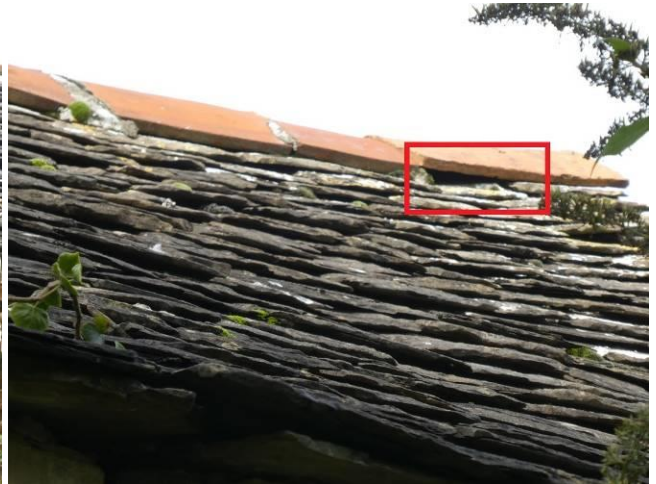
Photos 13 and 14 – Gaps under roof slates and clay ridge tiles [Sept 2019]
