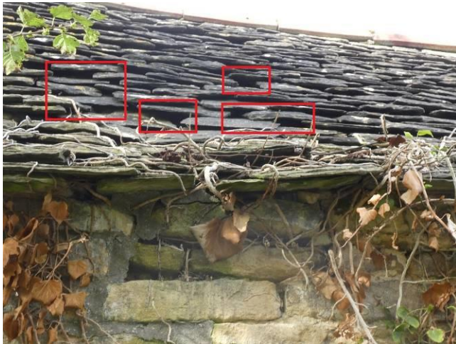
Photos 13 and 14 – Gaps under roof slates and clay ridge tiles [Sept 2019]
