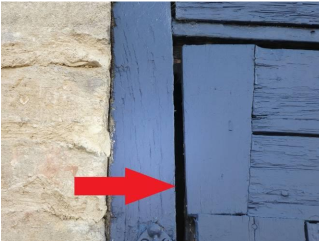
Photo 5 – Gaps at the side of the front elevation barn door, and, Photo 6 – Inside Lords Farm Barn [Sept 2019]
