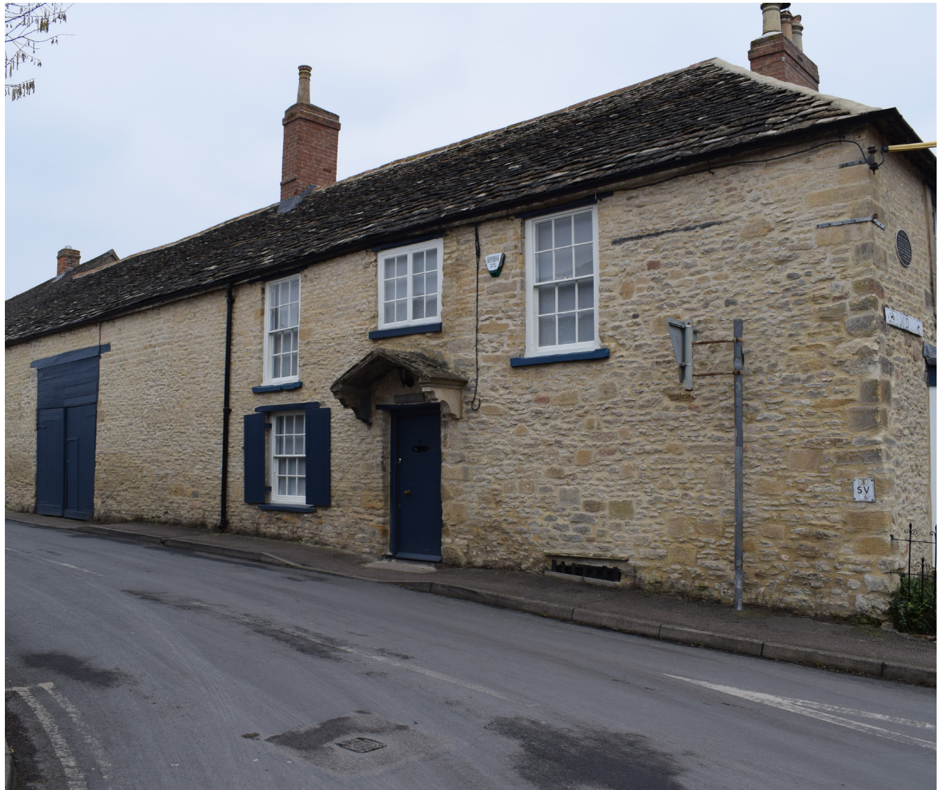
Fig 1: Front elevation of house and barn
