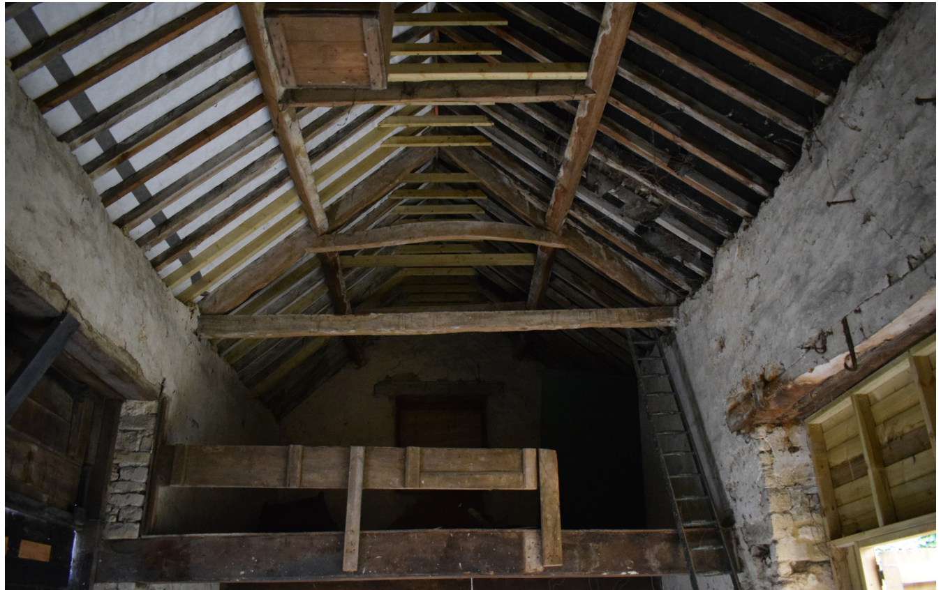
Fig 8: Double height space of barn with existing mezzanine level
