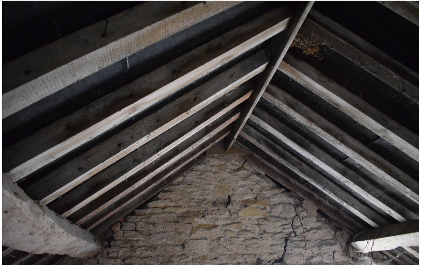
Fig 4: New roof structure in the stables building
