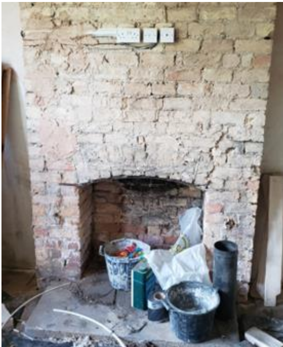
Fire Place 2 in the Living Room, no fire or surround present
