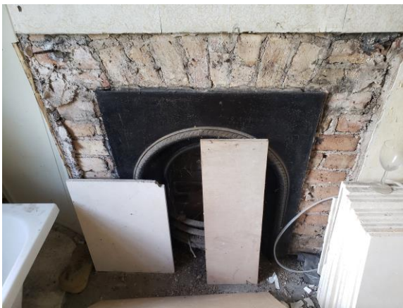
Fire place 8 in Bathroom
