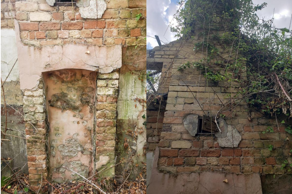
Fire place 7 in outbuilding 2. No fire or surround present. Sweeping door over fire place. Exposed brickwork within room suggests the entire original chimney was constructed from Gault brick. The top section is currently red brick.
