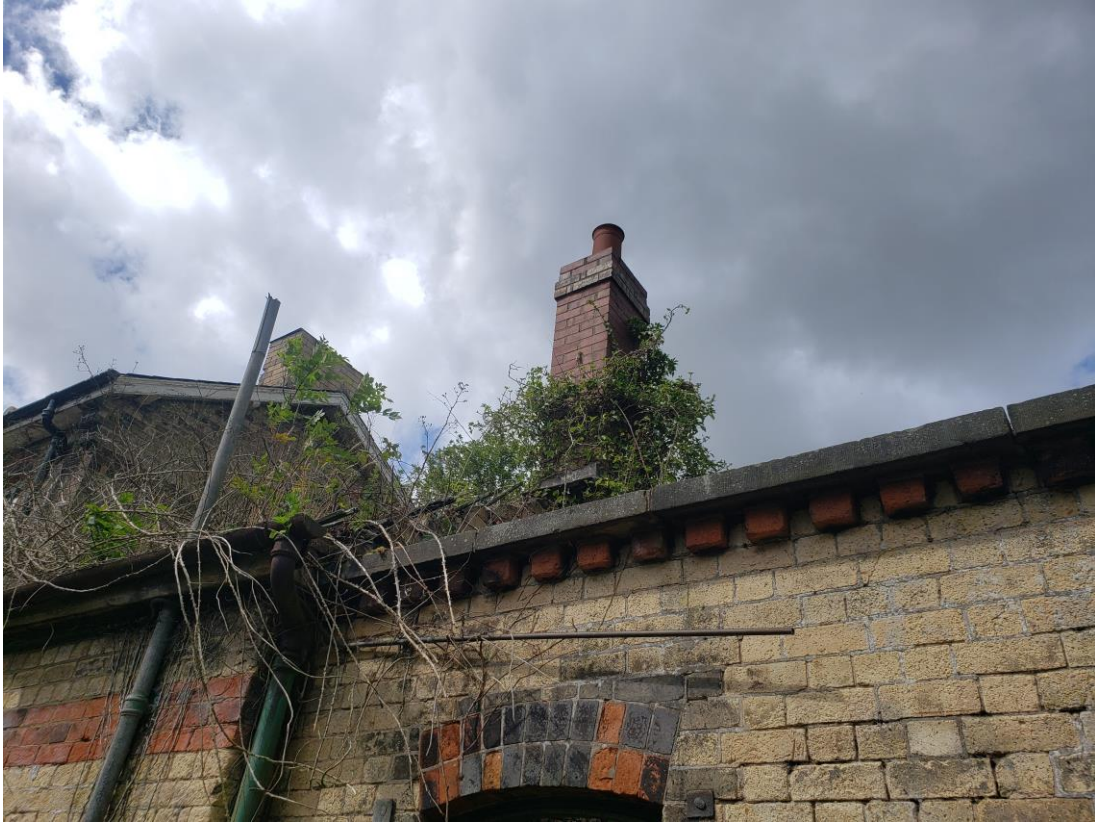
Current red brick chimney between outbuildings 1 and 2
