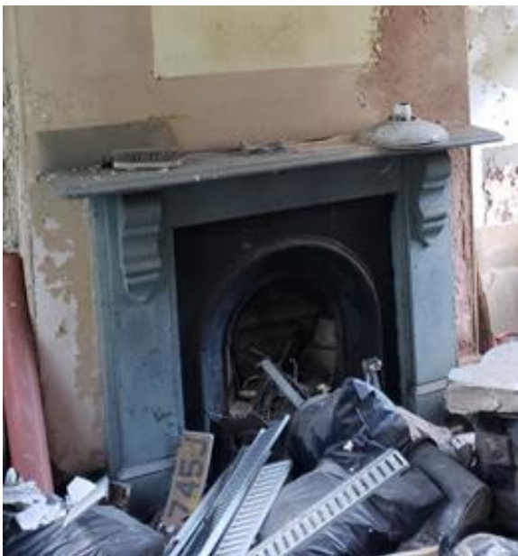
Fire place 4 in waiting area
