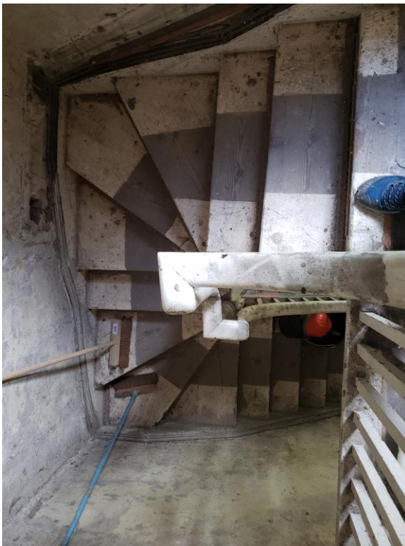
Winding staircase with original handrail
