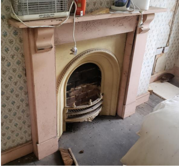
Fire place 9 in bedroom
