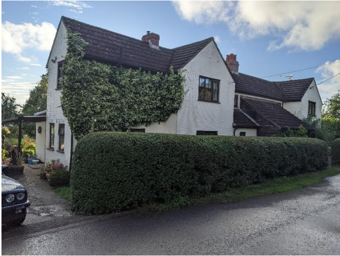
Photo 1 East and south elevations of the existing house
