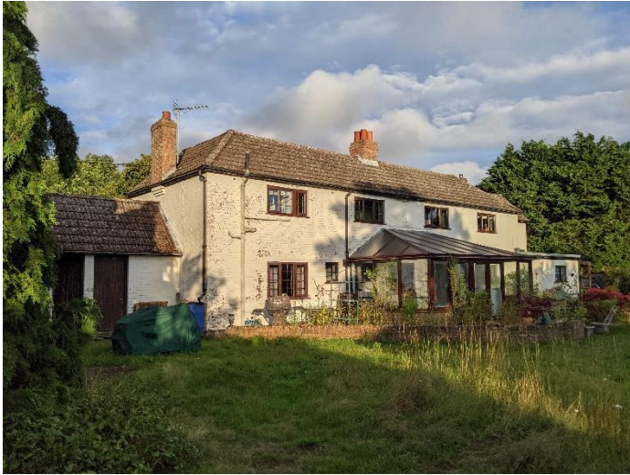
Photo 3 West and north elevations with area of short and longer grassland.
