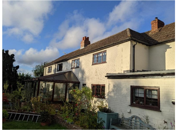
Photo 2 West elevations of the house
