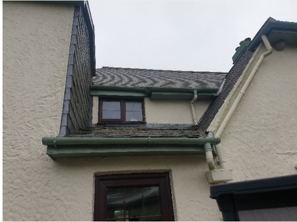
Middle section of east elevation
