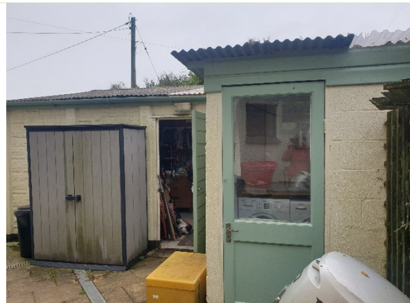
South-west elevation showing small built on utility room
