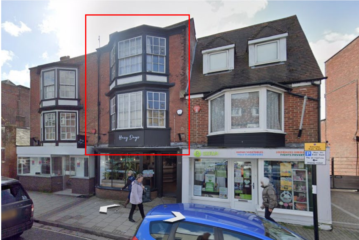
Figure 1 Front Elevation of Site, Google Earth
