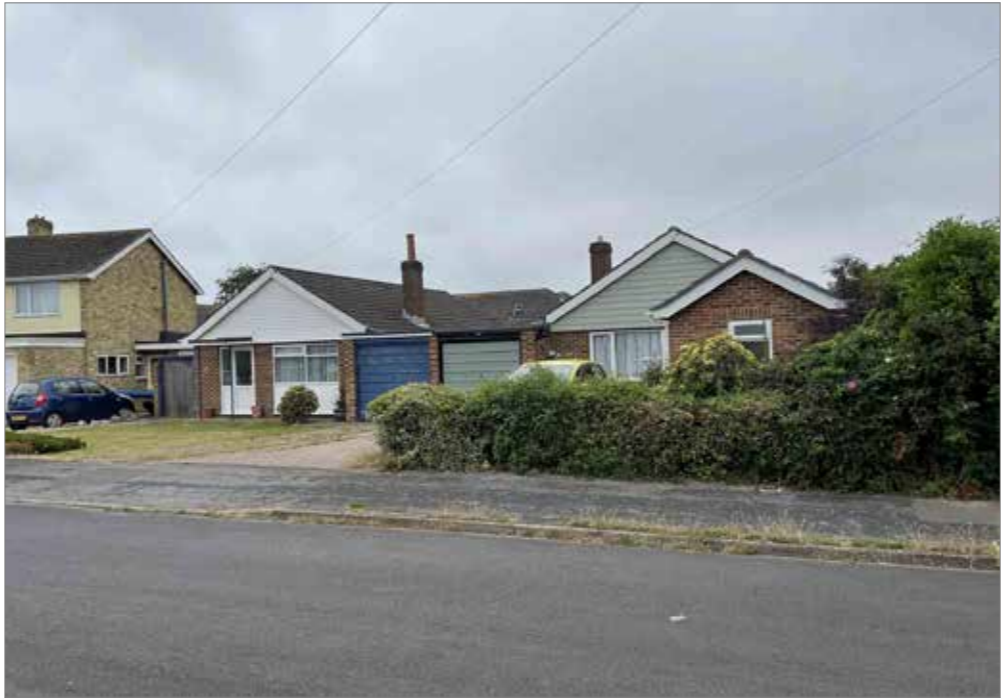
Fig 7-Alterations to neighbouring properties
