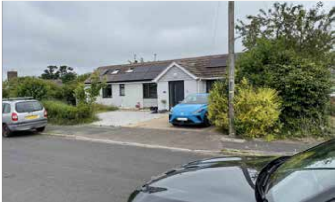
Fig 10-Alteration to neighbouring property
