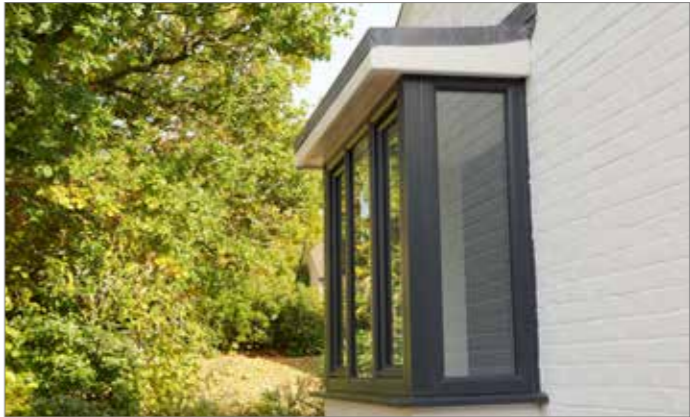
Fig 22-Bay Window ( White Framing)
