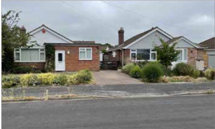
Fig 9-Alterations to neighbouring properties
