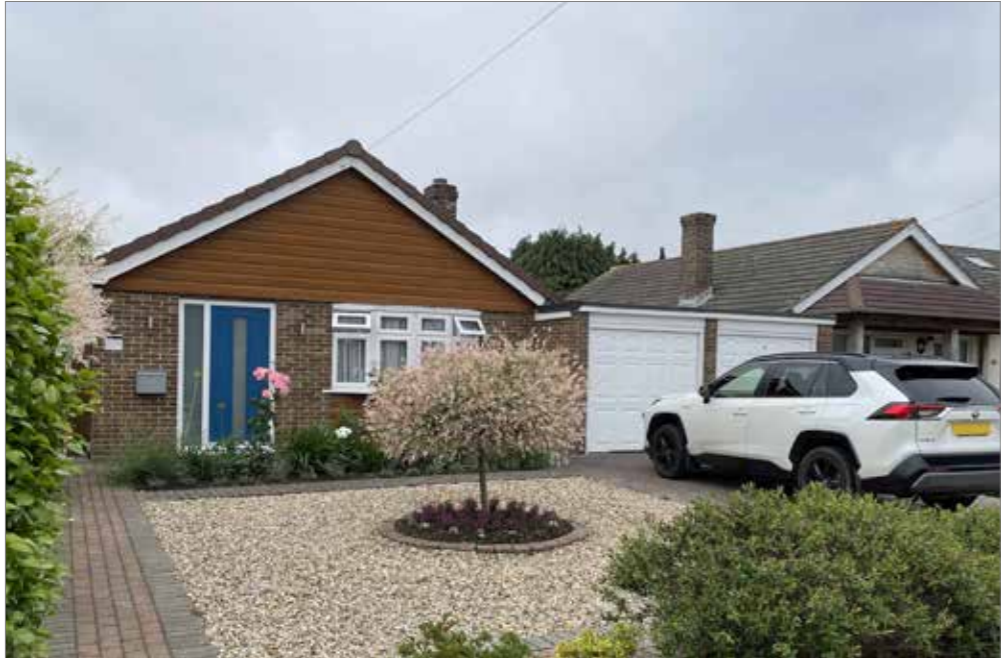
Fig 1-East Elevation seen from Pinewood Road
