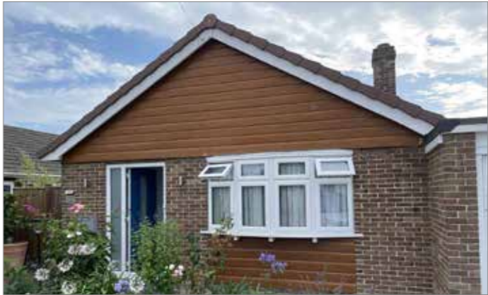
Fig 5-Detailed view of gable wall
