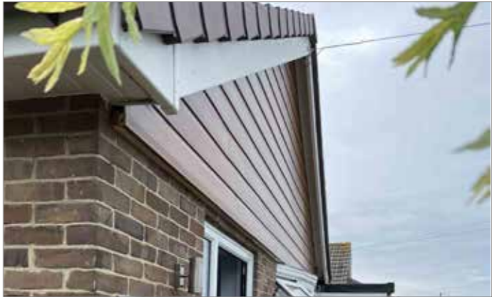
Fig 25-Eaves including closed boarding
