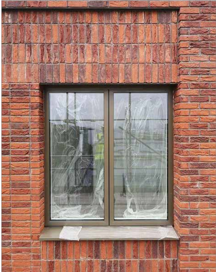
Fig 23-Feature soldier brickwork ( colour to match existing)
