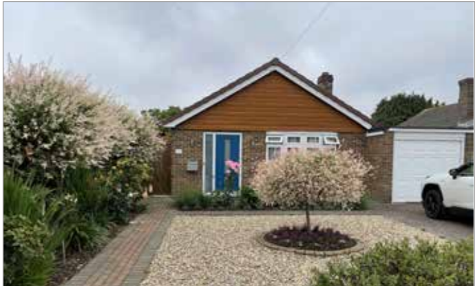
Fig 3-View of East Elevation
