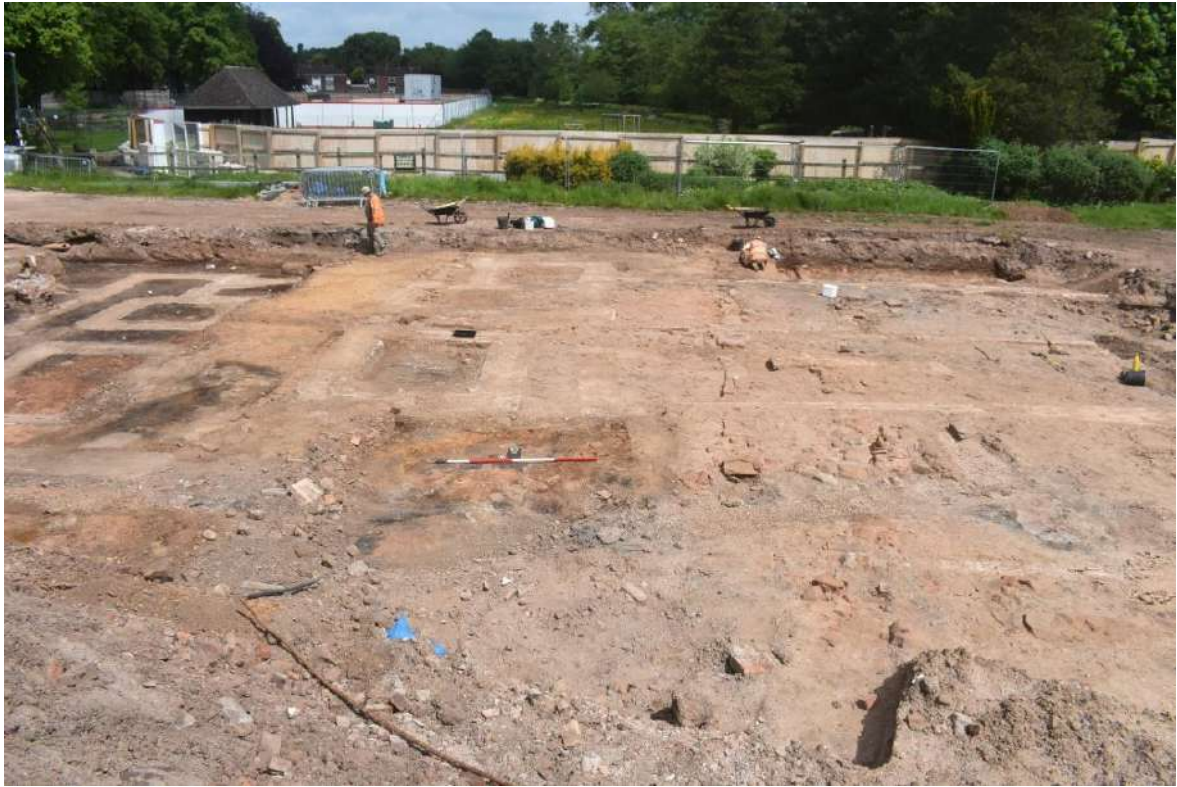
Photo 5 General view east across the southern buildings during cleaning showing the stone foundations running across the site and cut by the later pool foundations
