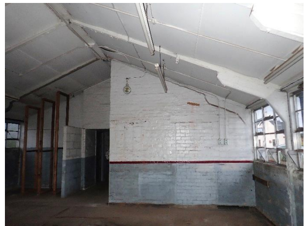
No loft area, roof lined
