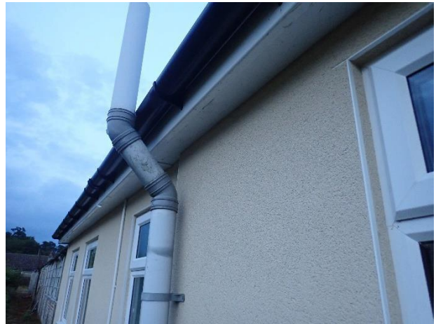
Soffits well sealed.
