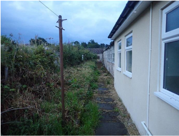
Cottage at west end, looking east.
