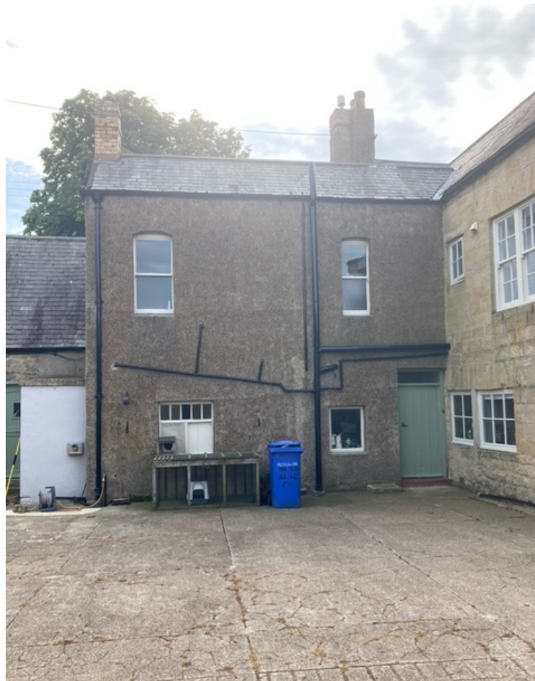
This shows the two current external finishes at Togston House
