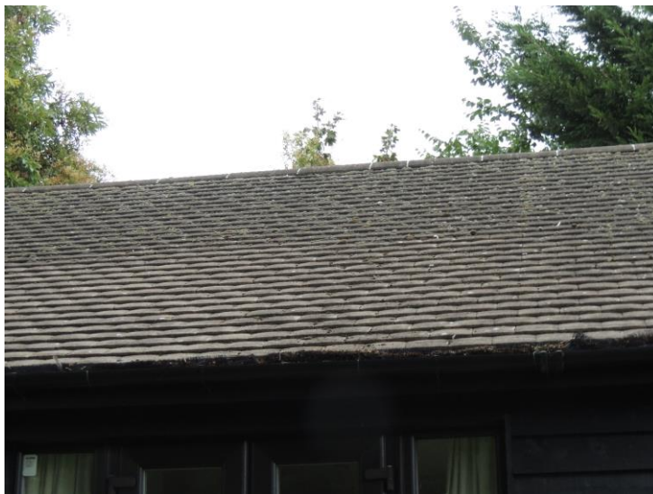
Photo 11: Note tight seal to roof tiles
