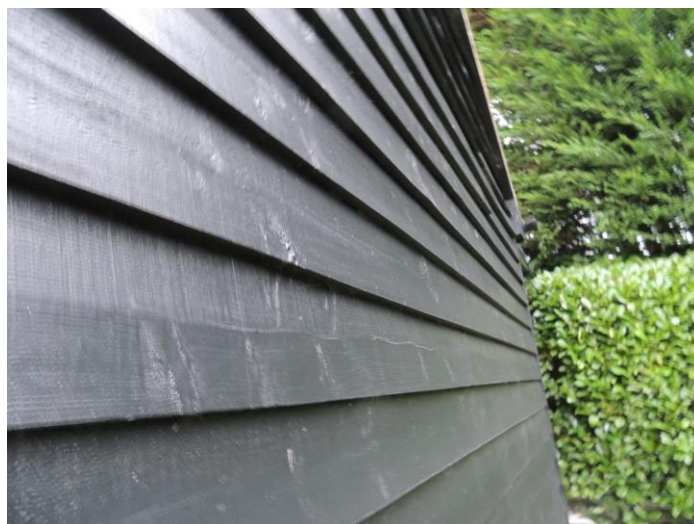
Photo 10: Note tight seal to wall cladding
