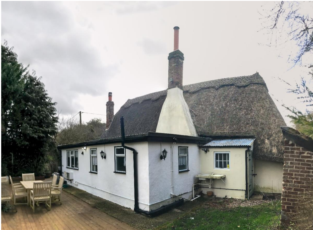
a - North corner of Forge Cottage showing the windows on the rear extension that are to be replaced
