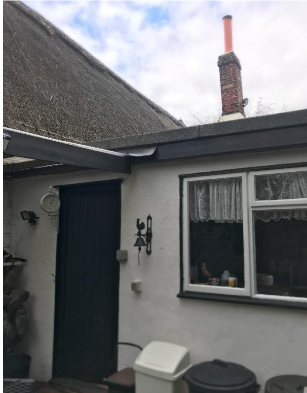
ç- External door to be replaced leading into kitchen
