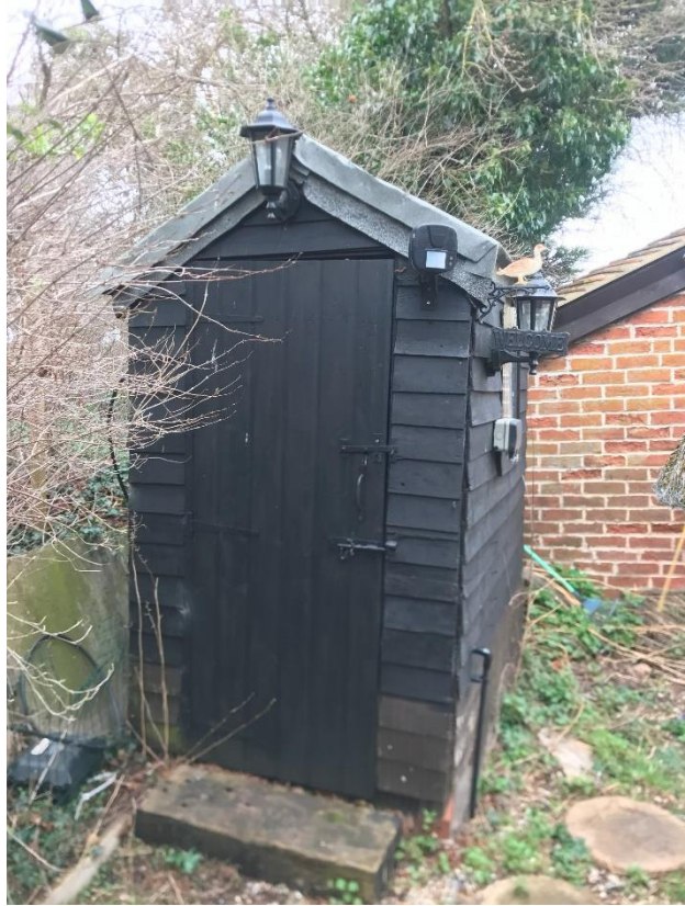
d - Timber framed shed like store that is to be demolished
