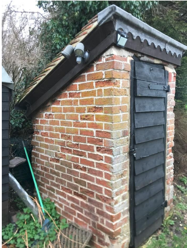
d- brick built store that is to be demolished
