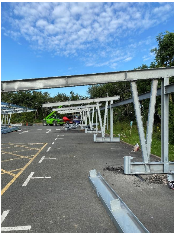
Dual bay monopitch Solarsense carport installed at Bicester Leisure Centre for Cherwell District Council
