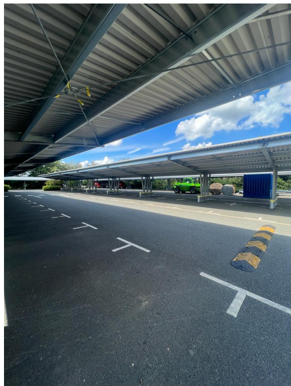
Dual bay monopitch Solarsense carport installed at Bicester Leisure Centre for Cherwell District Council
