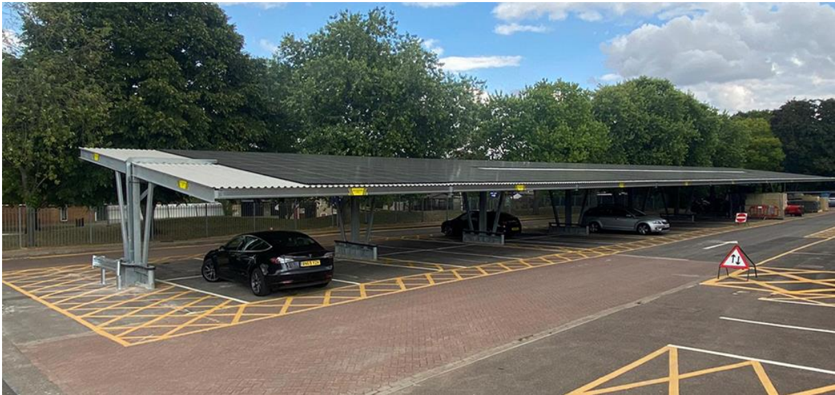
Dual bay monopitch Solarsense carport installed at Bicester Leisure Centre for Cherwell District Council
