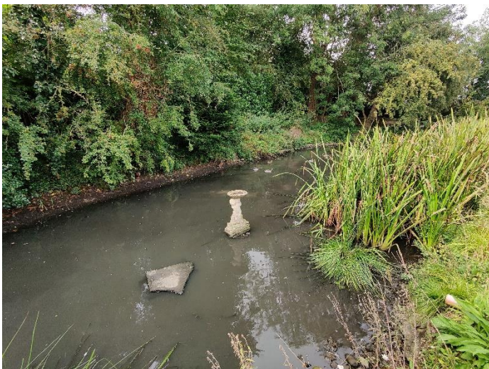
Photo 11 P1 viewed from the southeast
