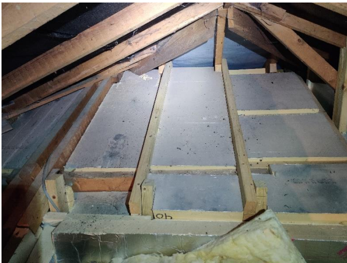
Photo 15 interior of the loft looking northeast
