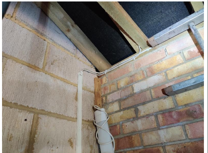
Photo 16 interior of the loft looking northwest
