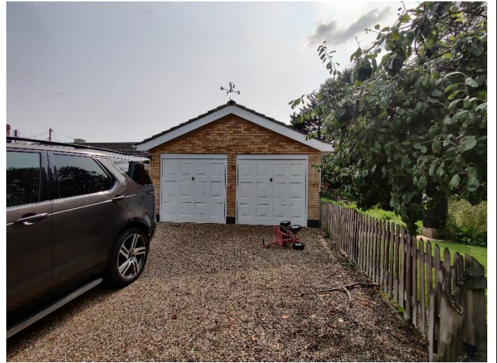
Photo 2 Existing garage off the west section of the northwest elevation
