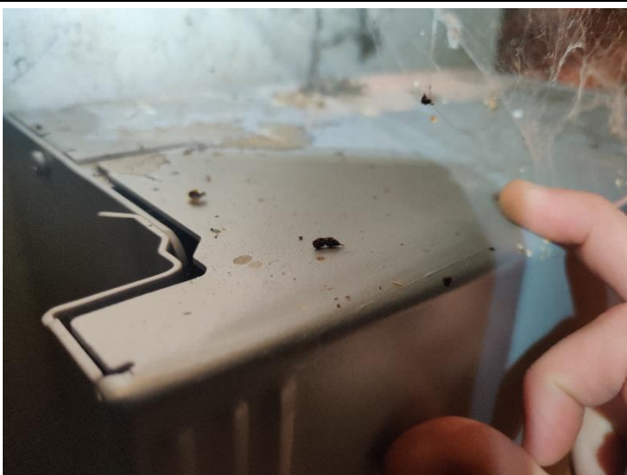
Photo 17 BLE dropping in the loft
