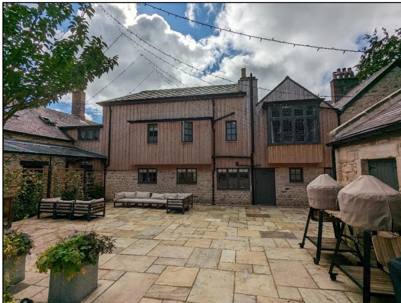
Plate 7. View of the courtyard. Rear of Main Building centre shot
