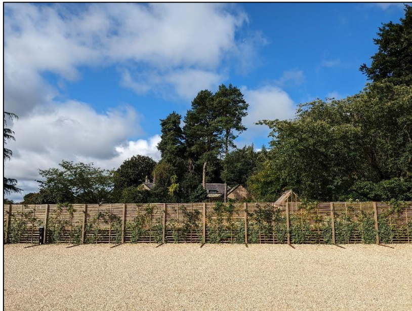
Plate 5. Car park with Farmhouse and ranges behind enclosure fence
