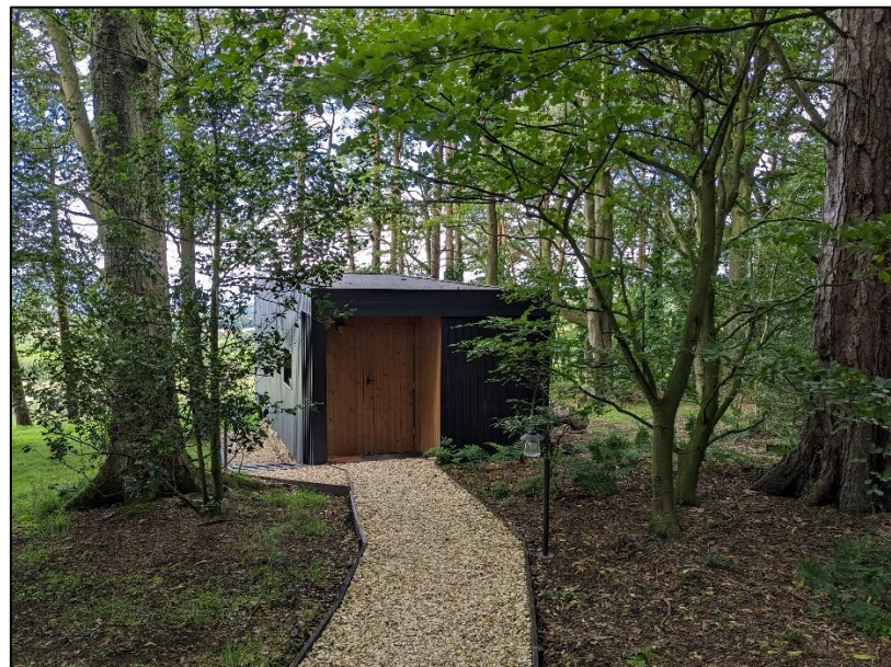
Plate 9. The Woodland Bridal Cabin Looking west
