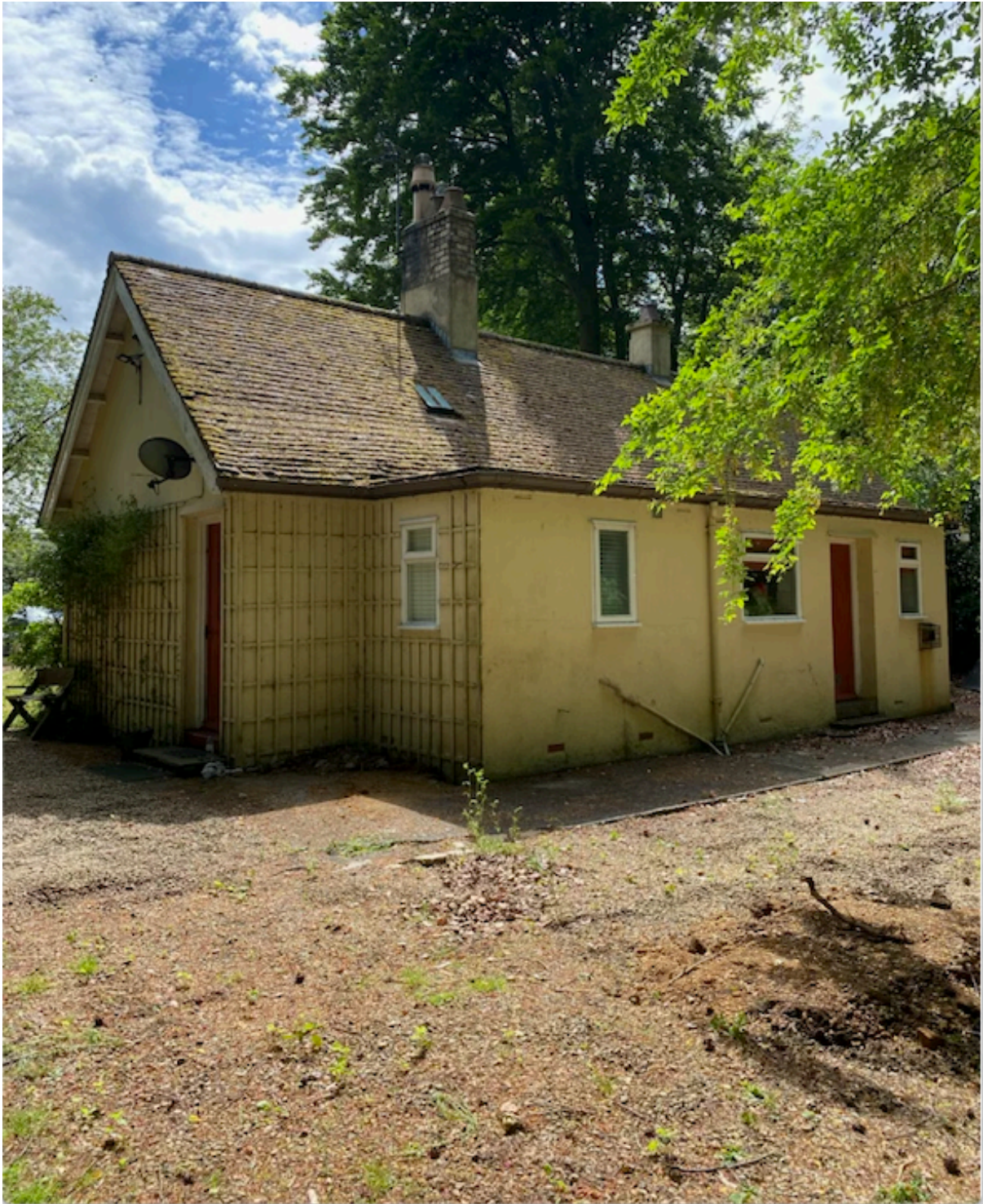
Image 1.2 - North-east (rear) elevation of the cottage – May 2020
