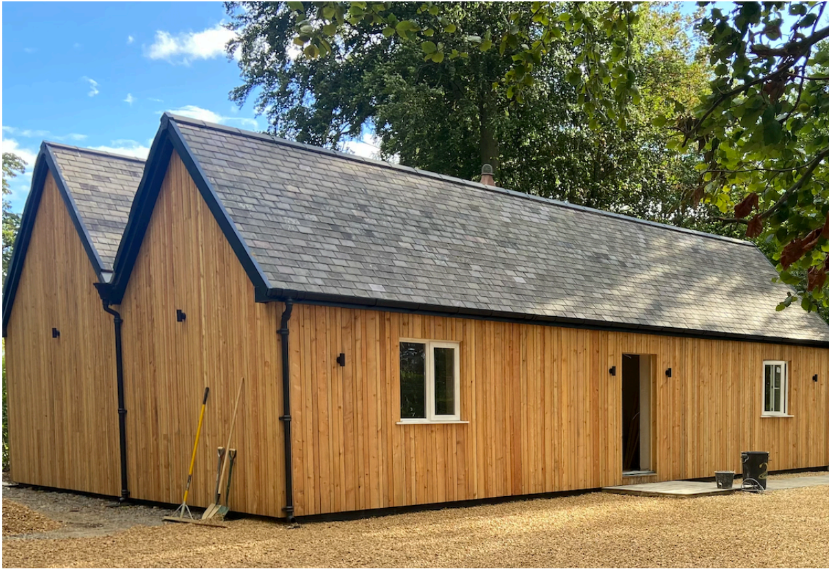
Image 1.3 – North-east (rear) elevation of the cottage – September 2022
