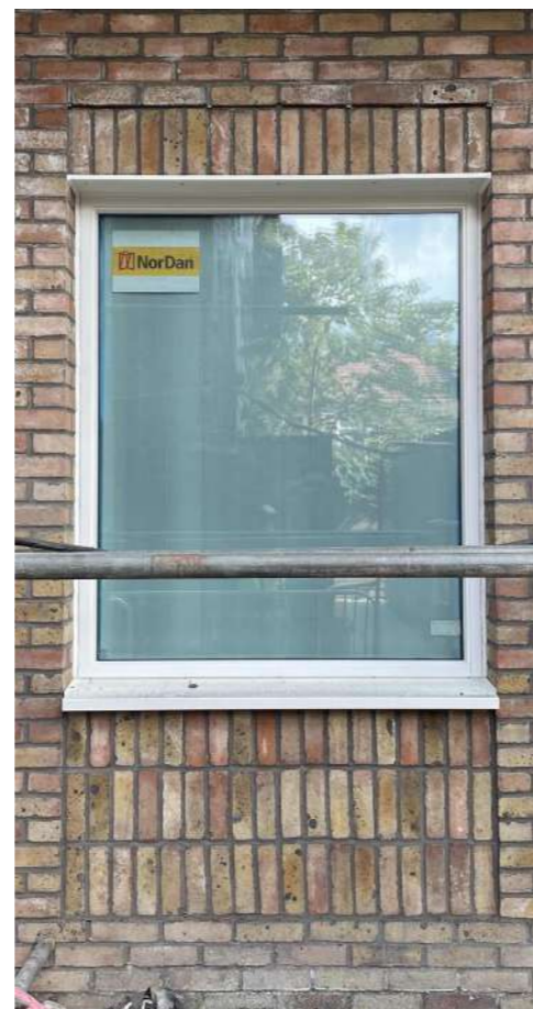
Fig.04 Window assembly benchmark with set back brick details
