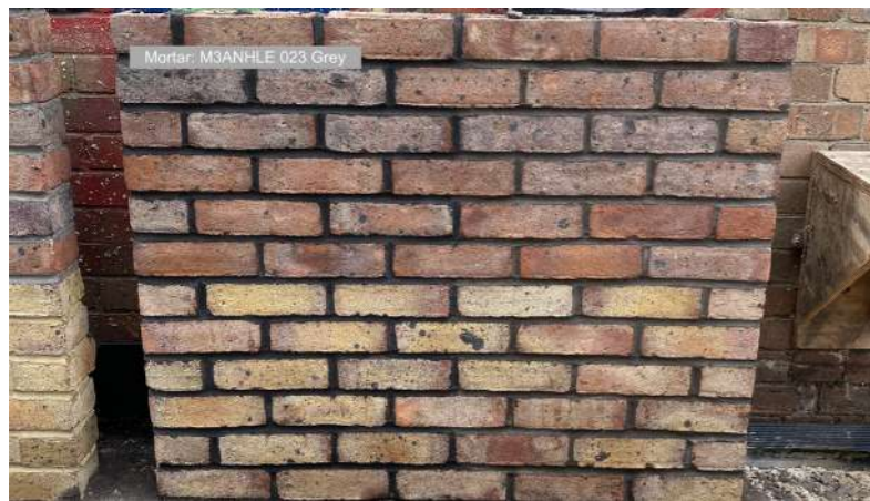
Fig.01 External brick mock ups
