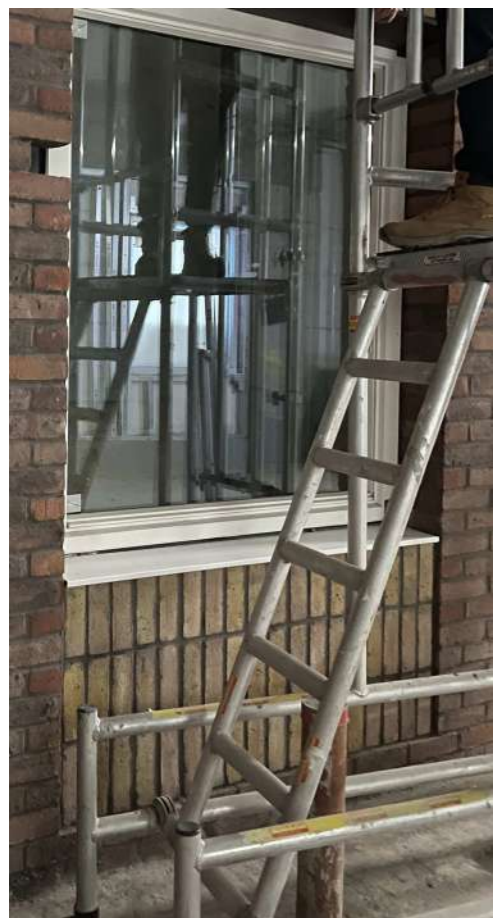
Fig.03 Window assembly mock-up showing window in brick wall with white sill and fascia
