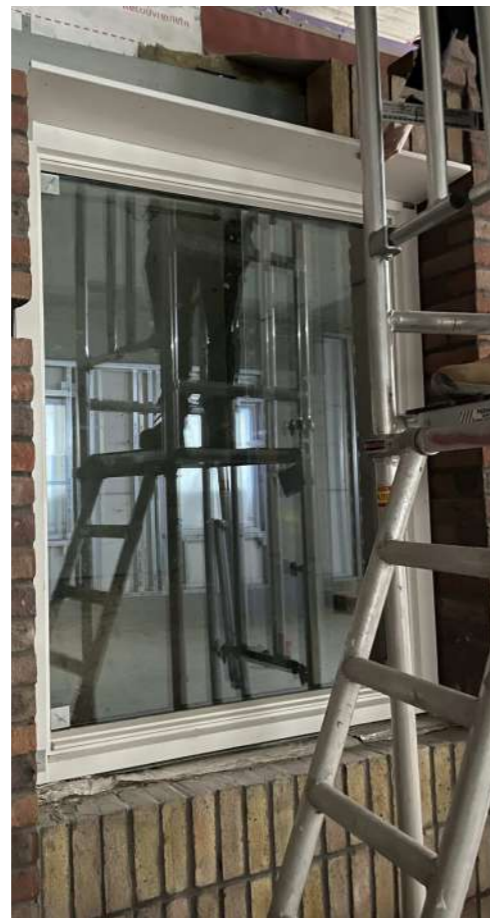
Fig.03 Window assembly mock-up showing window in brick wall with white sill and fascia
