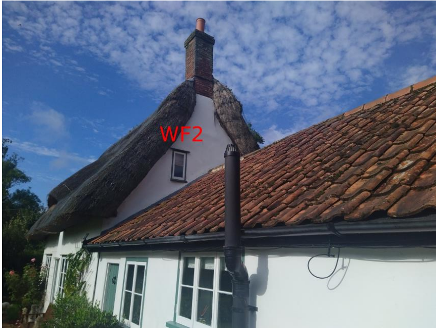
Side of dwelling (east)
