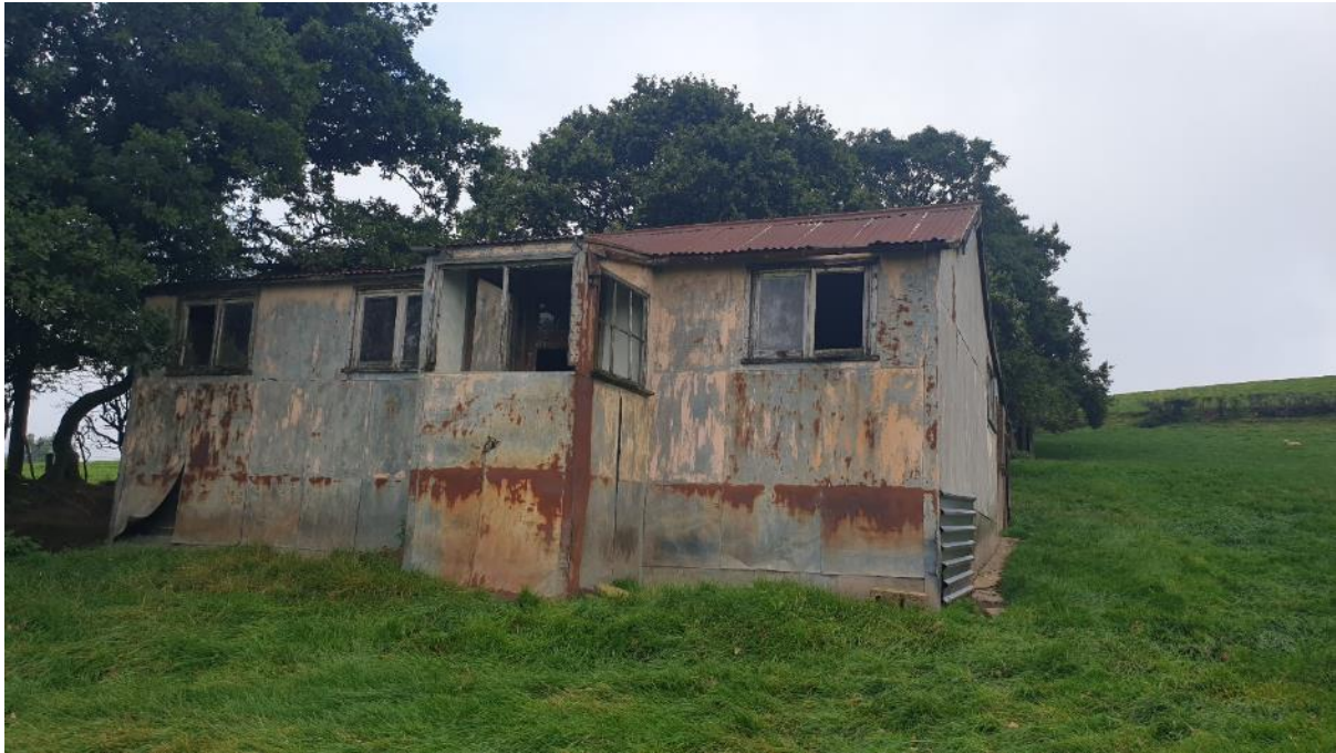
Photograph 1: Hele View from the front (south)
