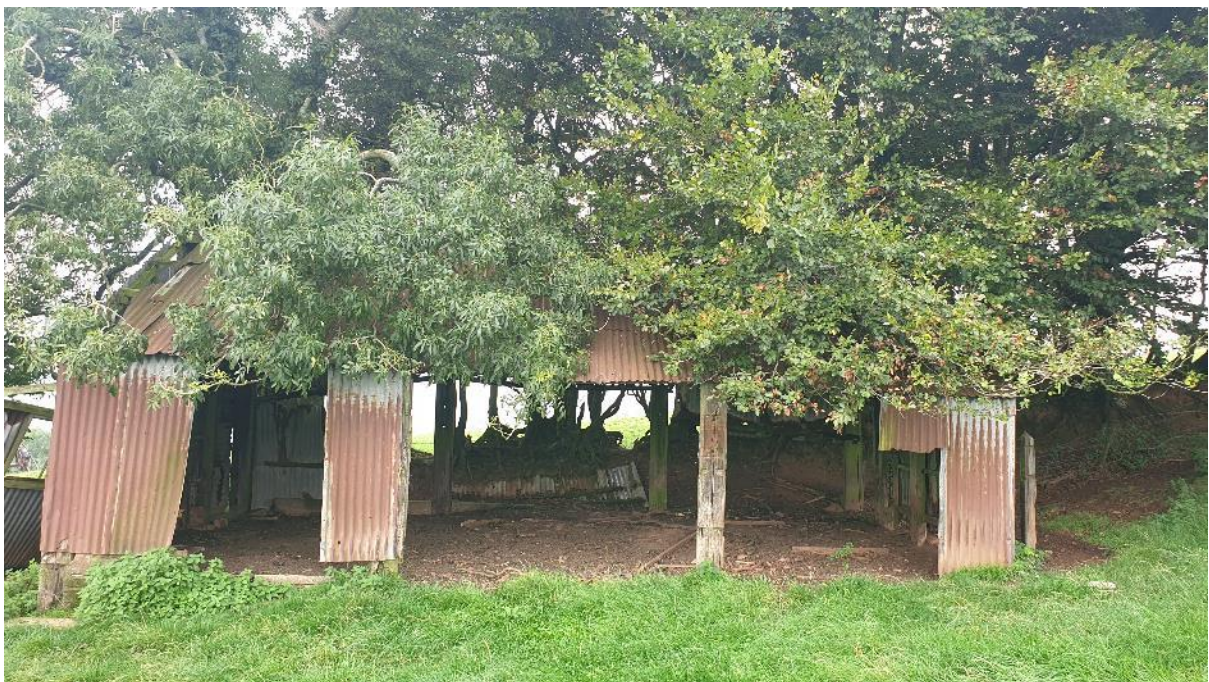
Photograph 5: Outbuilding 2 (to be converted into water storage/ancillary usage)
