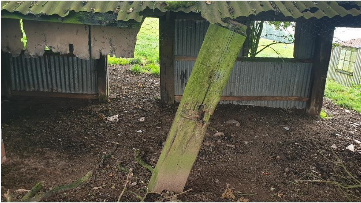
Photographs 4a & 4b: Outbuilding 1 (to be replaced with new annexe)
